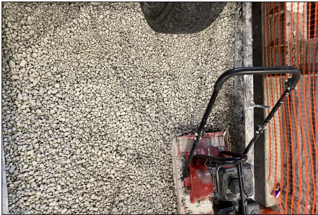
Figure 4.36 Compacted aggregate base course layer
