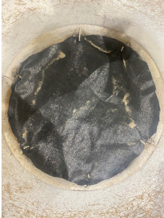
Figure 4.23 500X (GT) geotextile on compacted sand subgrade
