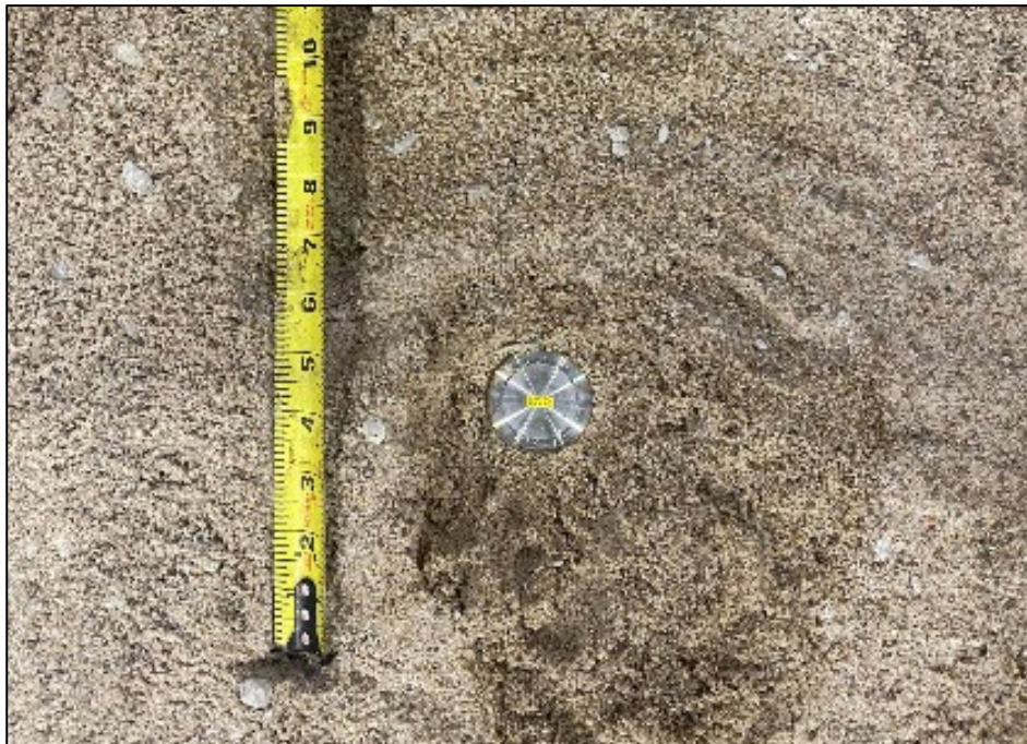
Figure 4.39 Pressure cell on compacted sand layer
