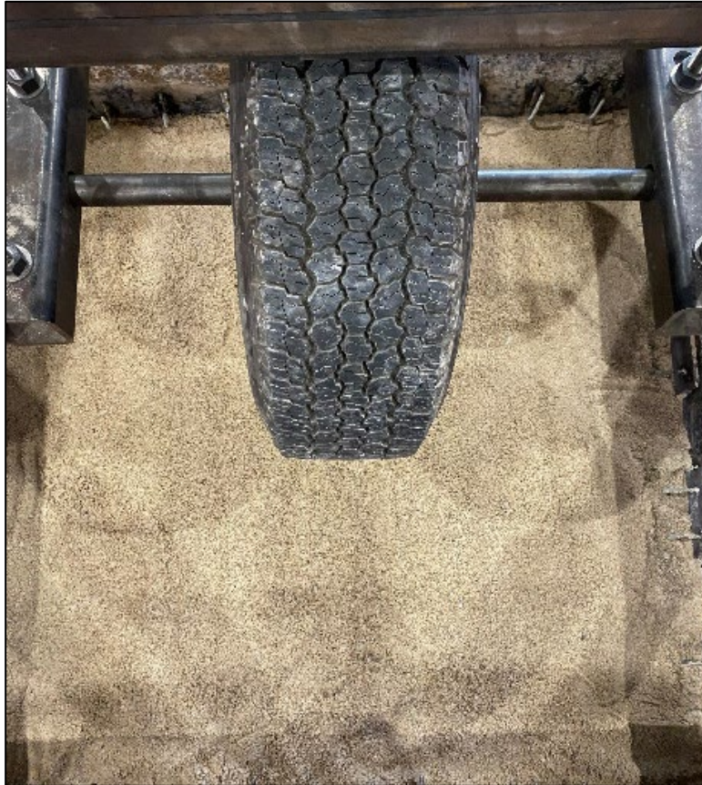
Figure 4.33 Compacted sand subgrade layer
