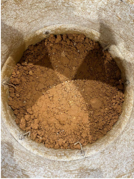
Figure 4.25 Compacted red shale subgrade layer
