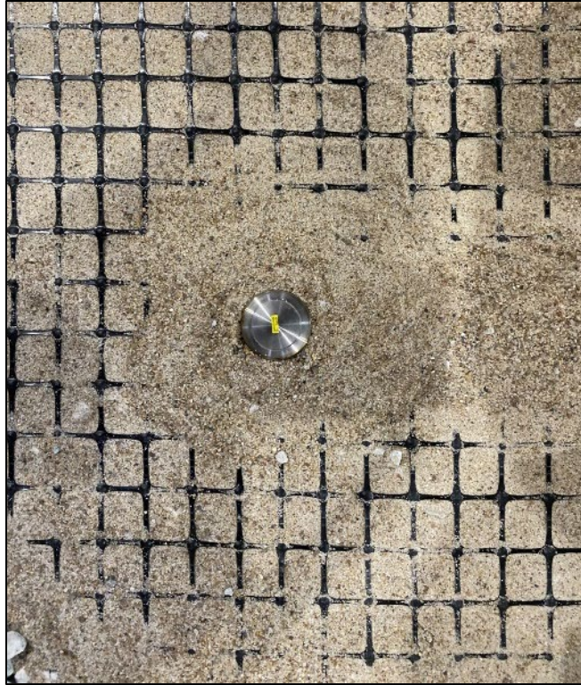
Figure 4.40 Pressure cell installed on top of geosynthetic location
