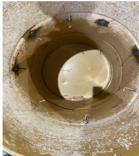
Figure 4.16 Hooks welded in steel barrel
