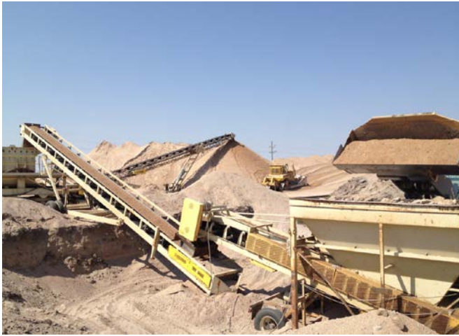
Figure 20. Aggregate Plant Site
