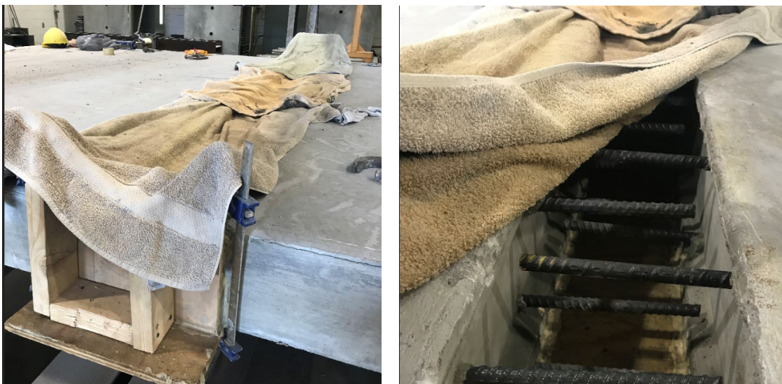
Figure 6.5 Field-scale connection preparation
