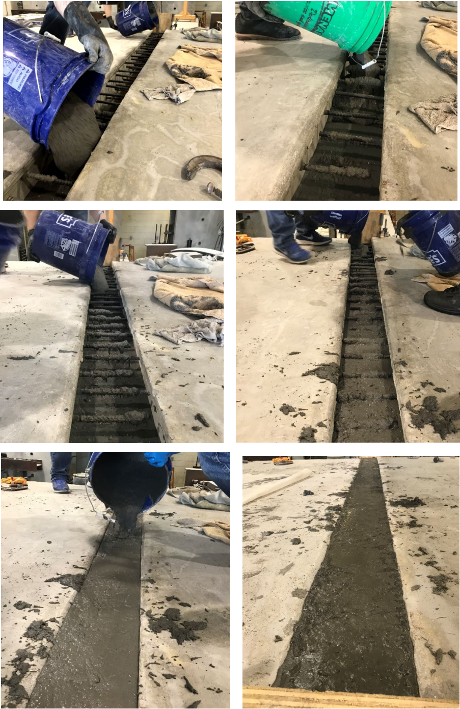
Figure 6.6 Field-scale connection UHPC placement
