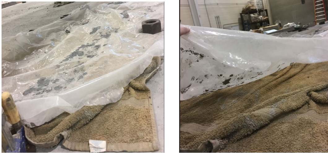
Figure 6.7 Field-scale connection UHPC curing
