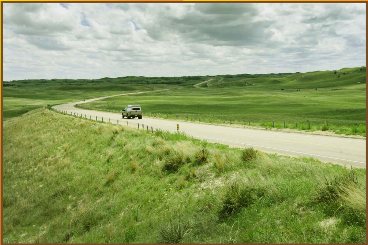
Hwy 83 south of Thedford.
