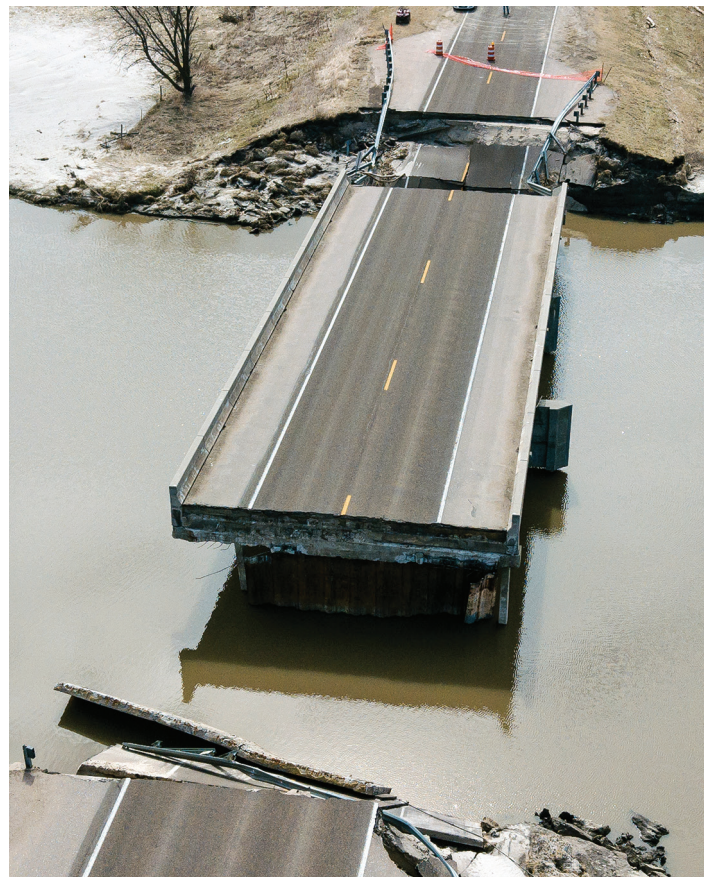
Flooding on the Loup River damaged the bridge on Hwy. 39 south of Genoa.
