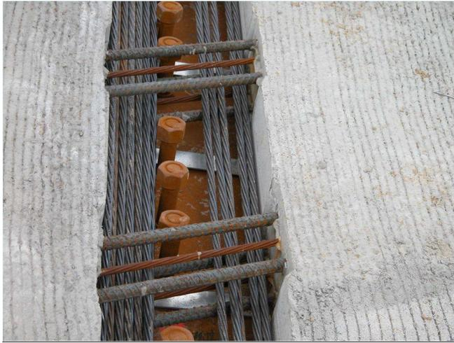
Figure 4.22-Post-tensioning Channel with Strands Pulled through
