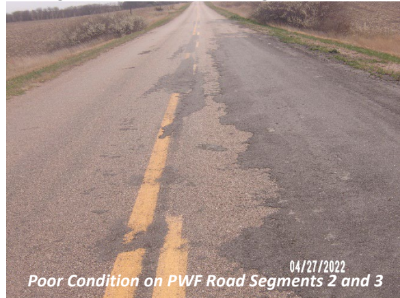
Figure 8: Extensive Road Patching on PWF Road
