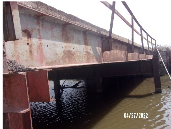
Figure 12: Bridge Substructure and Abutment
