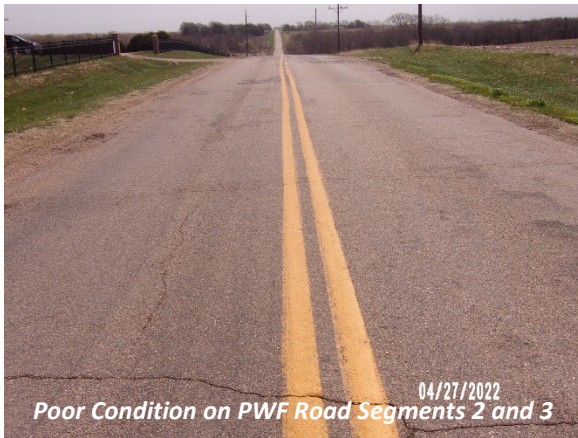
Figure 5: Areas of Extensive Pavement Cracking and Rutting on PWF Road
