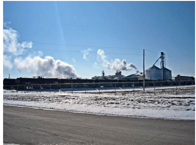
Railroad access line for an ethanol plant.
