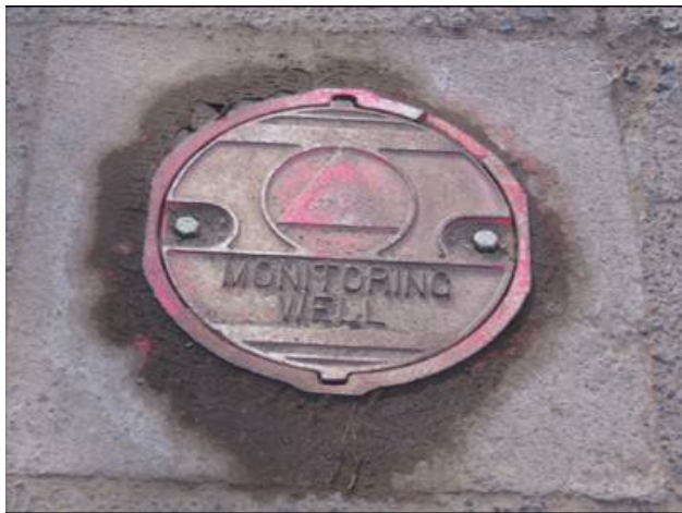
Flush mount monitoring well.
