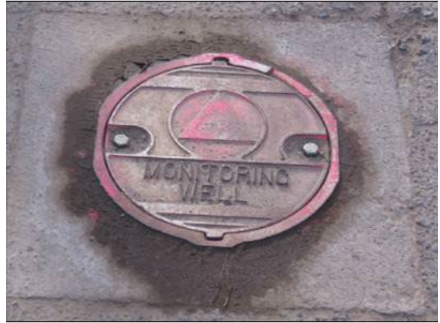
Typical in-ground monitoring well.
