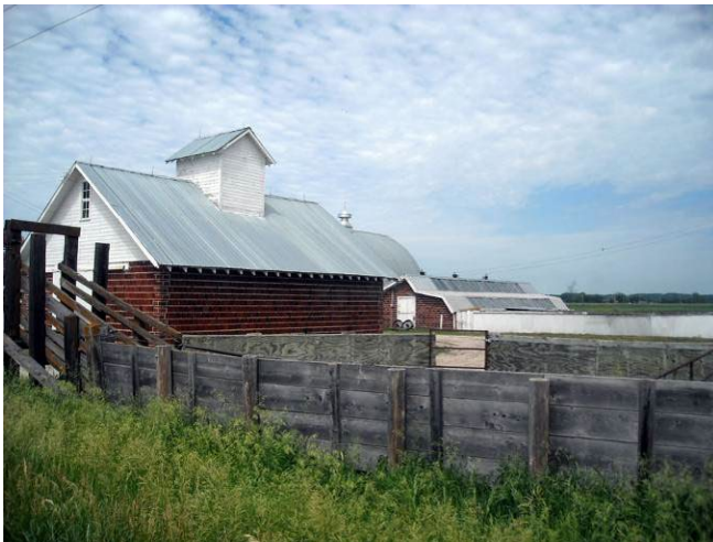
Paint on old buildings may contain heavy metal-based paint.
