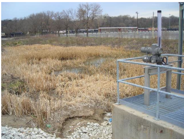
Detention pond at an agricultural chemical manufacturing facility.
