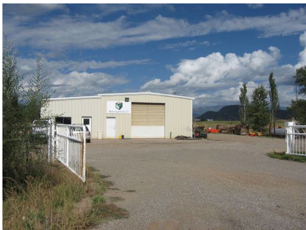
Two 55-gallon drums (to the right of garage) associated with property adjacent to highway right-of-way. One drum is tipped over.
