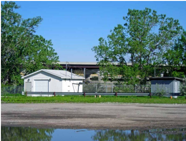
Typical groundwater remediation sheds.
