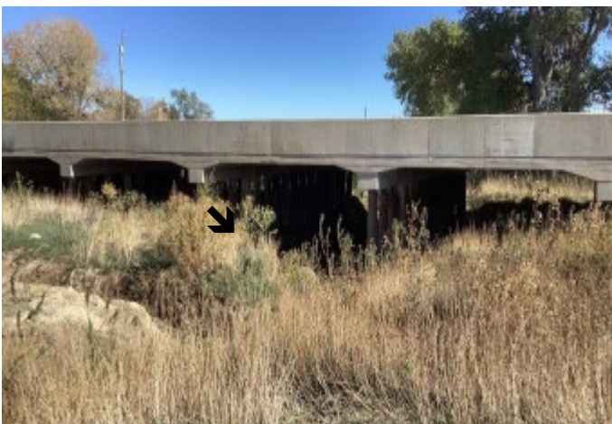
Profile of a bridge during inspection.
