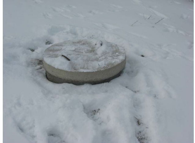
Residence with probable septic system.
