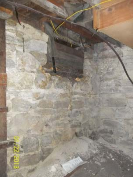
123 South 3 rd Street, coal chute
