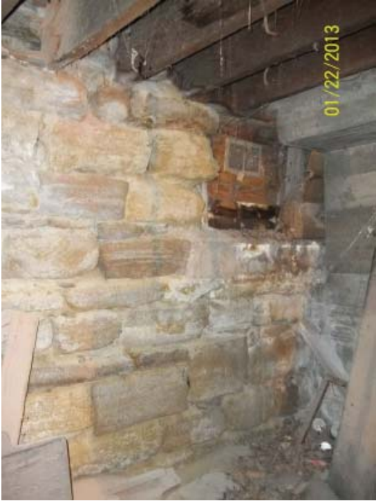
Lutheran Family Services, coal chute
