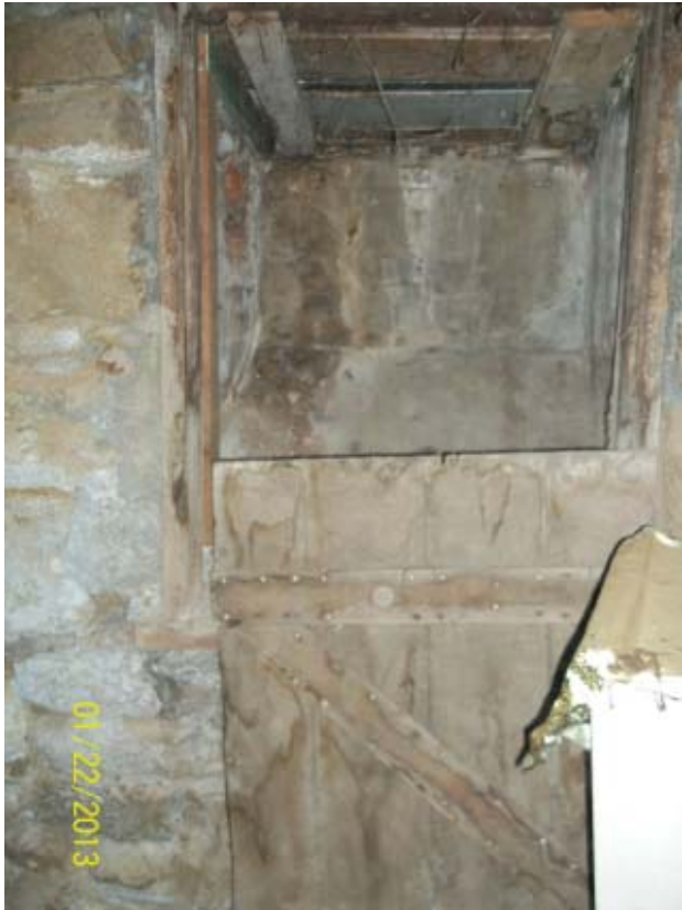
117 North 3 rd Street, Coal Chute
