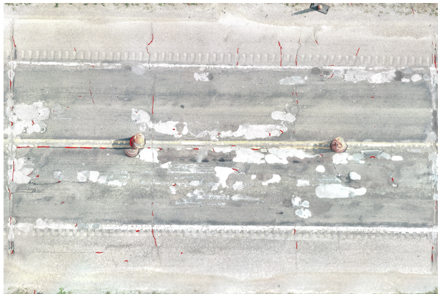
Fig. 3.15. Stitched image of asphalt overlaid concrete deck for bridge S075 17062
