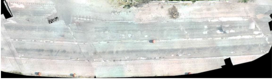
(a) Stitched UAV image collected on asphalt overlaid concrete deck
