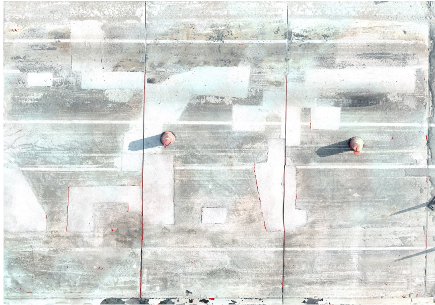
Fig. 3.16. Stitched image for Bridge S075 17062 collected on repaired concrete deck
