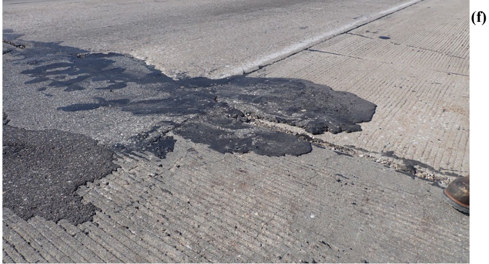
Figure A.10 (continued) Current state of repair material installed at location 3
