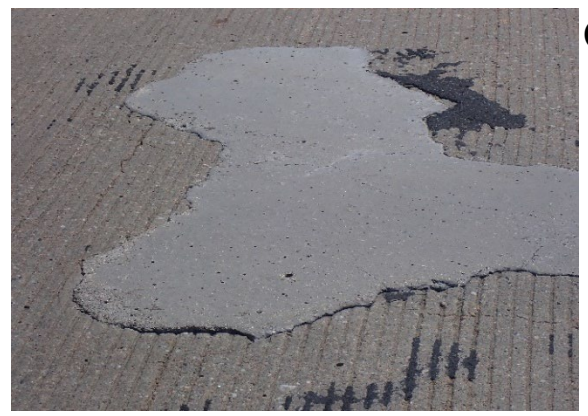
Figure Appendix A.18 Current state of repair material installed in location 2
