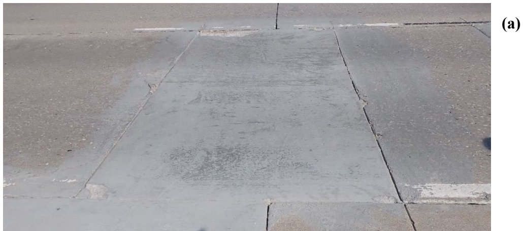
Figure Appendix A.11 Current state of repair material installed at location 4
