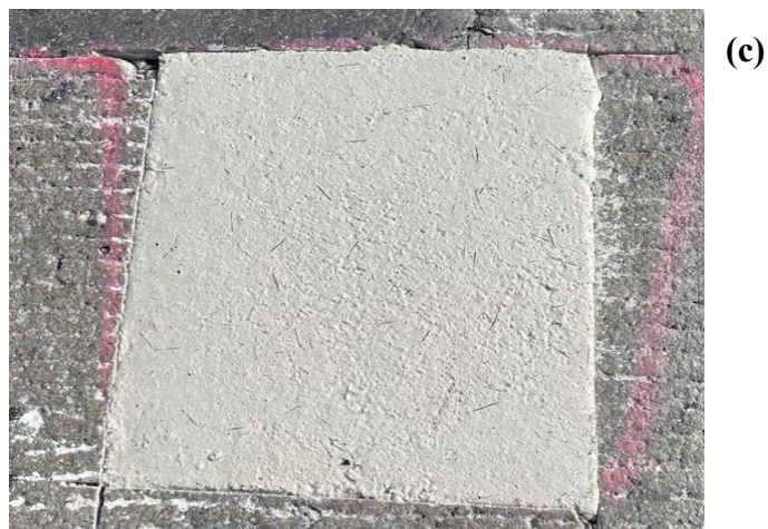
Figure Appendix A.5 Current state of repair material installed at location 5
