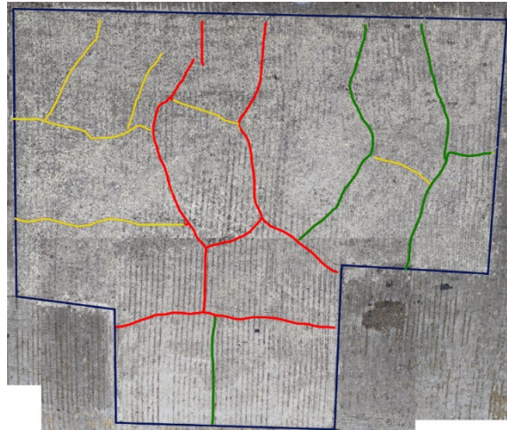
Figure Chapter 2.4 Example of field inspection of prebagged material in an ongoing study
