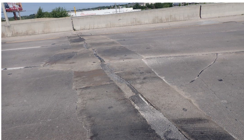
Figure A.12 (continued) Current state of repair material installed at location 5
