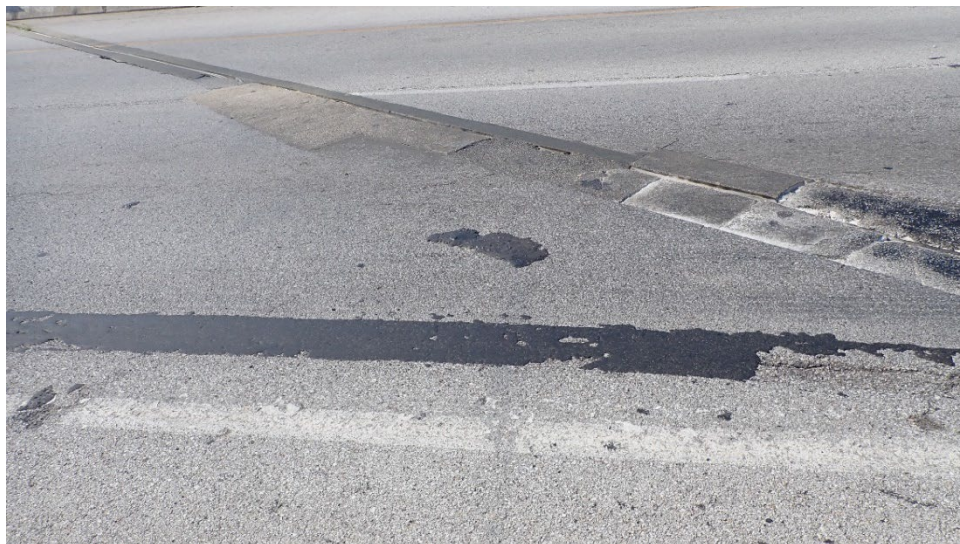
Figure Appendix A.8 Current state of repair material installed in location 1
