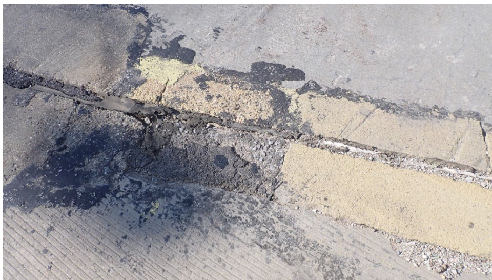
Figure Appendix A.10 Current state of repair material installed at location 3
