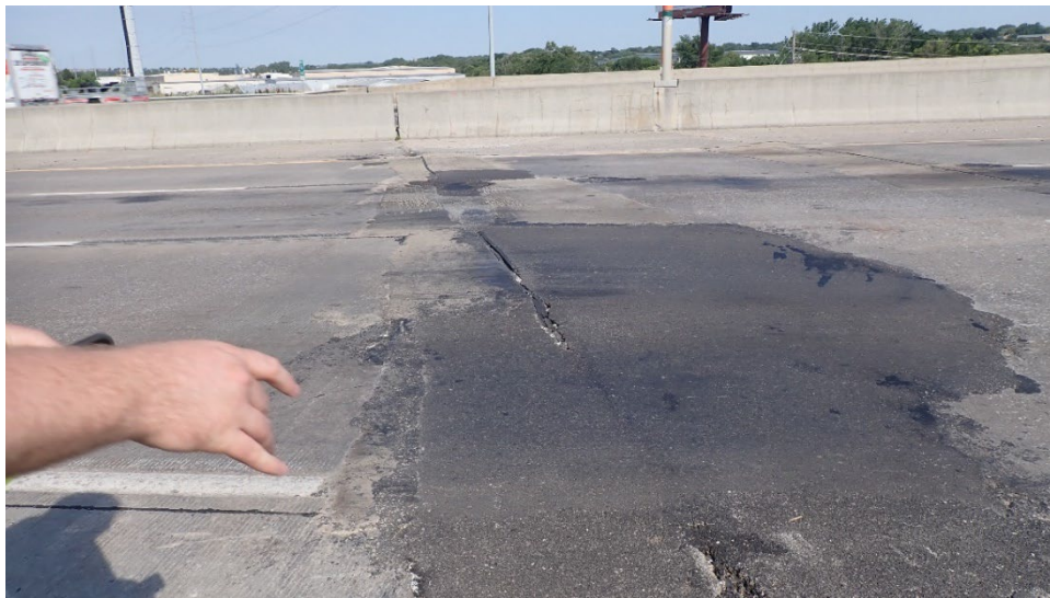
Figure Appendix A.12 Current state of repair material installed at location 5
