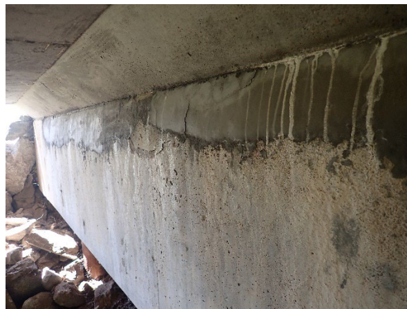
Figure Appendix A.17 Current state of the repair material installed at location 1
