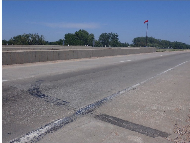
Figure A.21 (continued) Current state of the repair material at location 4
