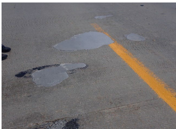
Figure Appendix A.18 Current state of repair material installed in location 2
