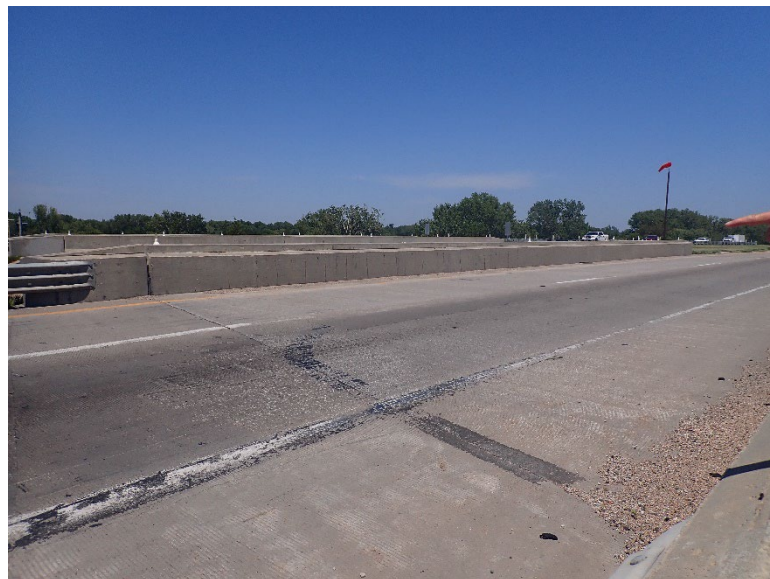
Figure Appendix A.21 Current state of repair material installed at location 4
