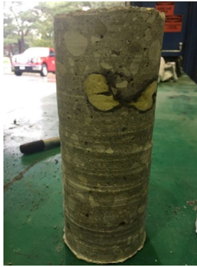
Figure 2.18 Slab 3 - Core 12 (Oblong Void)
