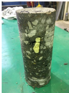
Figure 2.17 Slab 3 - Core 8 (Large Void)
