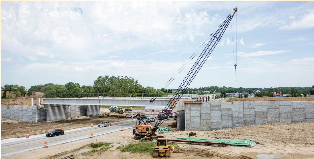
Construction on Nebraska City Project
