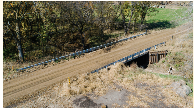
County Bridge Match Program site in Thayer County
