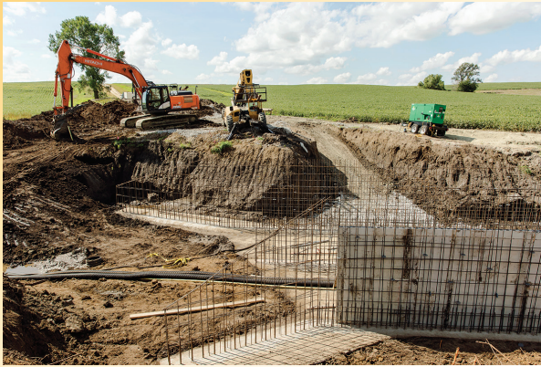
County Bridge Construction Site West of Palmyra
