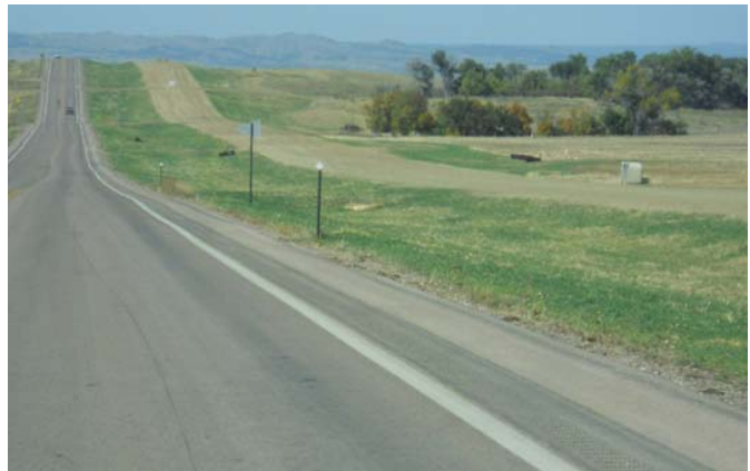
Figure 3.20 – Work beginning on widening US 385 to four-lanes north of Oelrichs, SD
