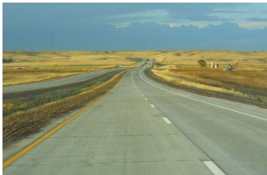
Figure 3.12 – NE 71, north of Kimball, already widened to 4 lanes
