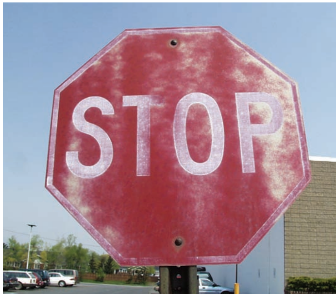
Figure 13 - Sign in poor condition
