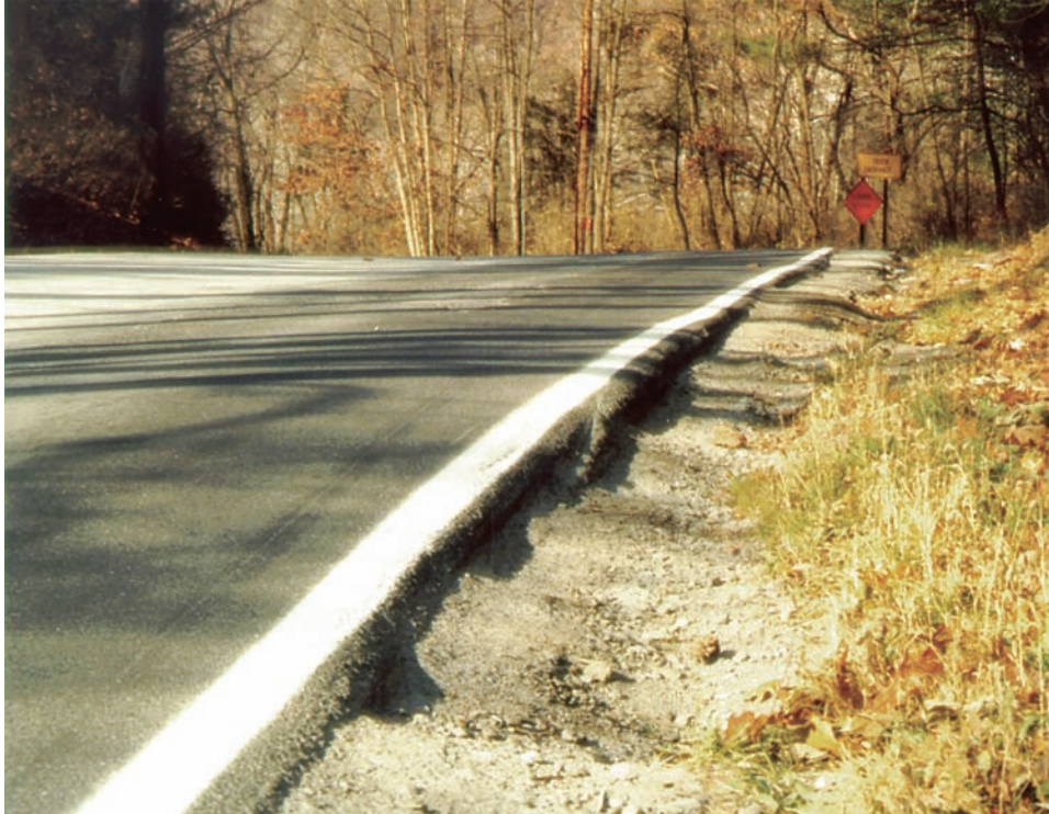
Figure 17 - Edge drop-off
