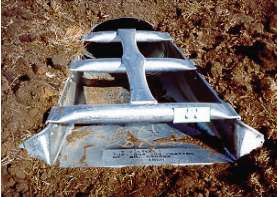
Figure 18 - Culvert safety end section
