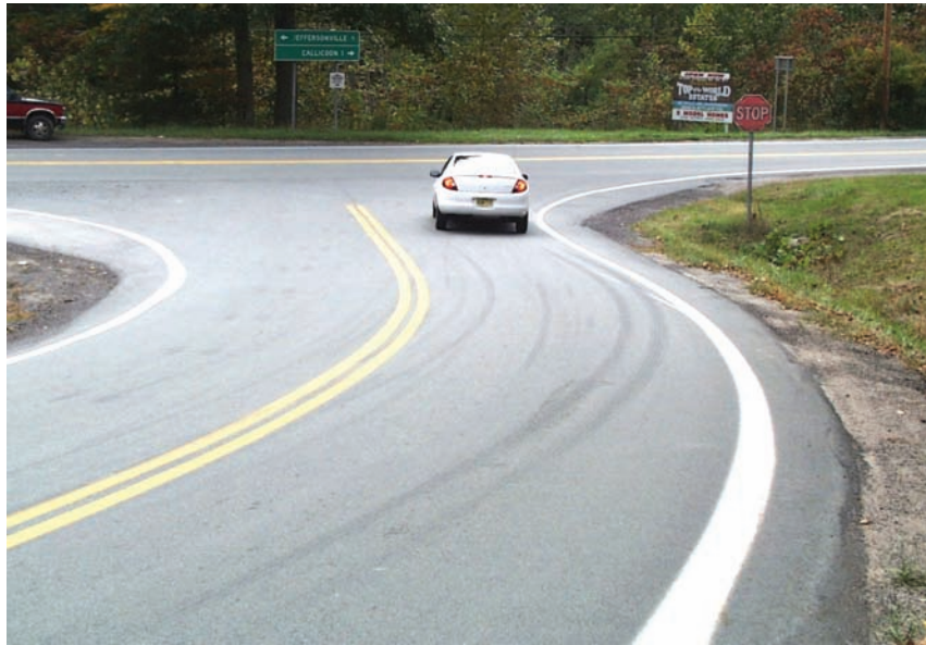
Figure 7 - Skid marks often indicate problems
