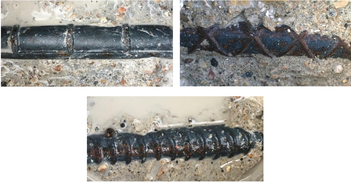
Figure 8: Typical Reinforcement Condition in Bridge S075 17596
