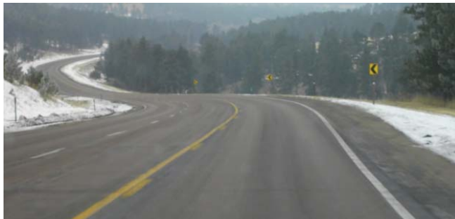
Figure 2.21 – US 385 Through the Nebraska National Forest, Three-Lane Highway with Climbing Lane for the Southbound (Uphill) Direction.
