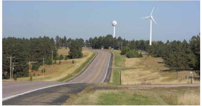
Figure 2.20 – US 385, Three-Lane Highway Through the Nebraska National Forest, Approximately Ten Miles South of Chadron at Mile Marker 157.
