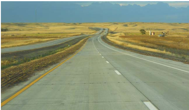
Figure 2.13 – NE 71, Four-Lane Highway Kimball to Scottsbluff
