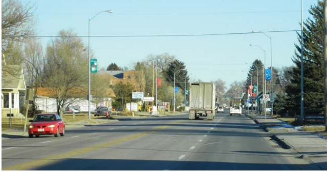
Figure 2.17 – US 26, Four-Lane Highway Through Mitchell, NE
