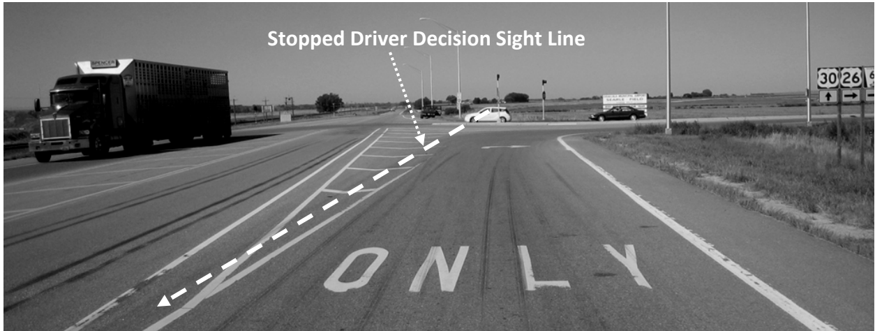
FIGURE 6 Site 7, Tapered-Type ORTL at the Intersection of Hwys US-26 & US-30 in Ogallala, NE
