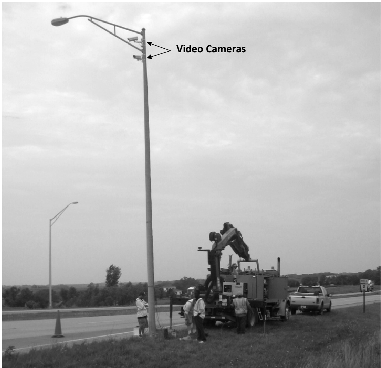
FIGURE 31 Field Assembly at Site 1 During Installation
