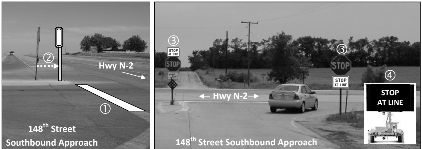
FIGURE 28 Preliminary Suggestions to Improve Stopped Driver Location Choice on Southbound Stopped Approach at 148 th Street.
