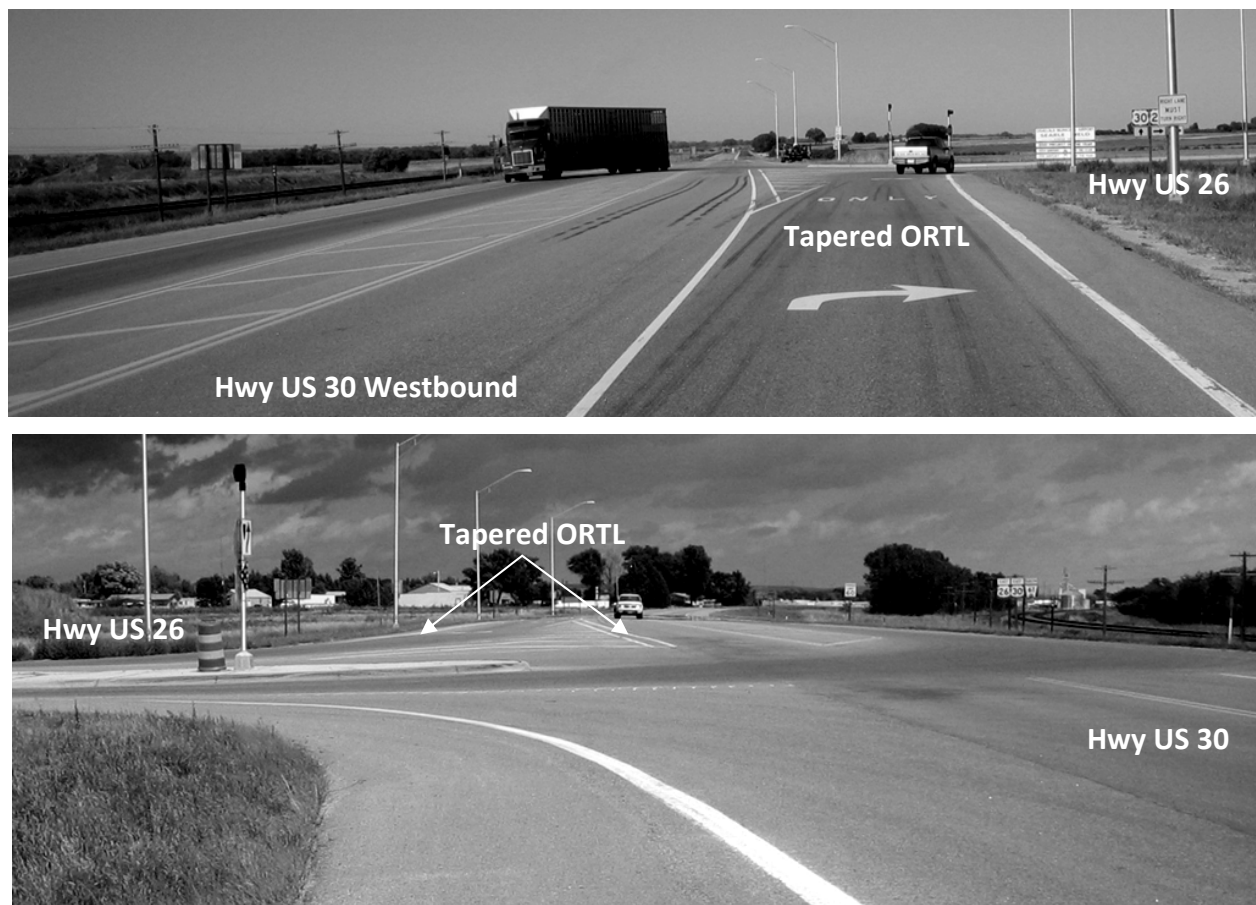
FIGURE 47 Site 7, Hwys US-26 and US-30 west of Ogallala, Nebraska
