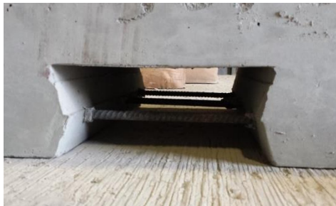
Figure 3.03: Initial Design Proposed Panel Trough.
