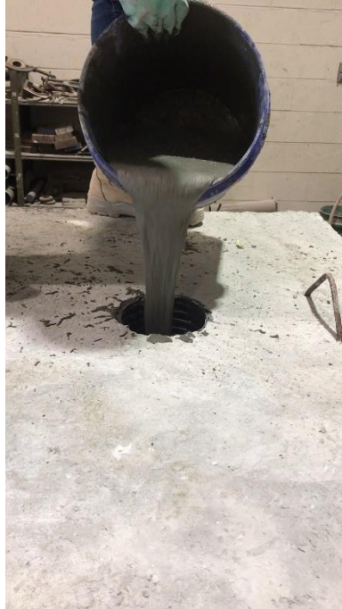
Figure 4.034: UHPC Casting for UHPC#2 Specimen.
