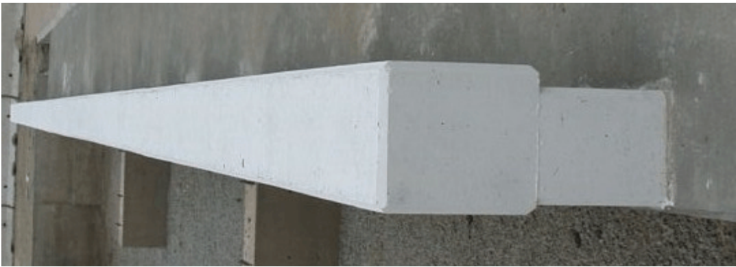
Figure 13. Open Concrete Bridge Rail
