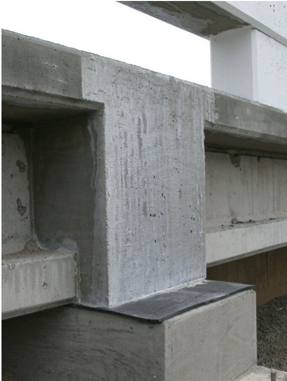
Figure 11. Lateral Stiffener End Caps at Bent Joints
