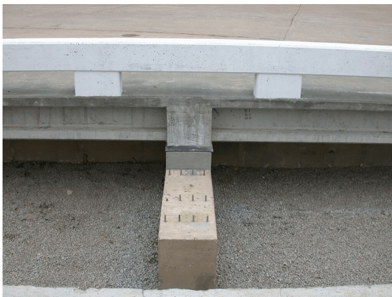
Figure 14. Open Concrete Bridge Rail
