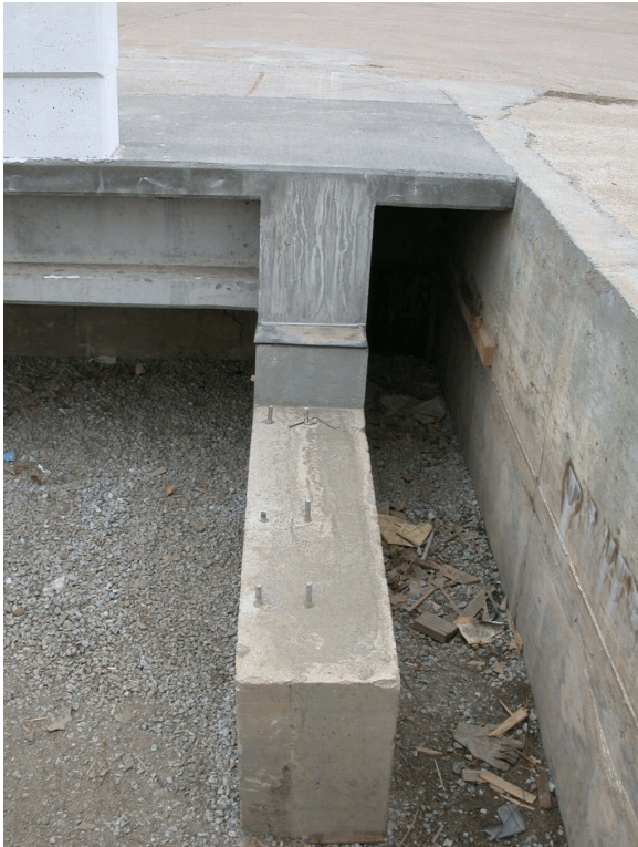
Figure 10. Lateral Stiffener End Caps at Upstream and Downstream Abutment Joints
