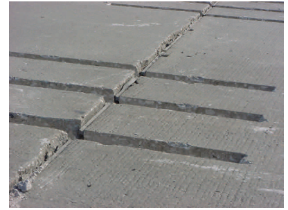
Picture 1.1: Removed pavement for new dowel bars.
