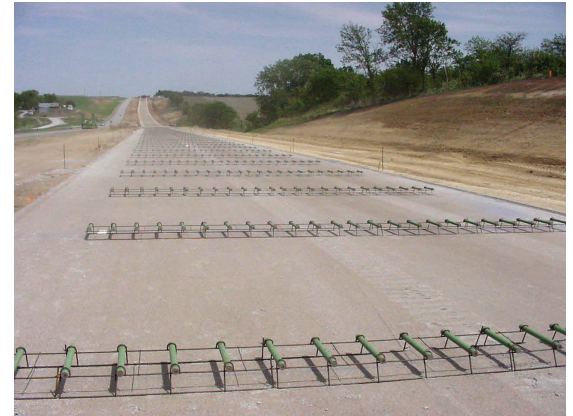
Dowel bars placed on chairs ready for paving. (Photo compliments of Lieska Halsey)
