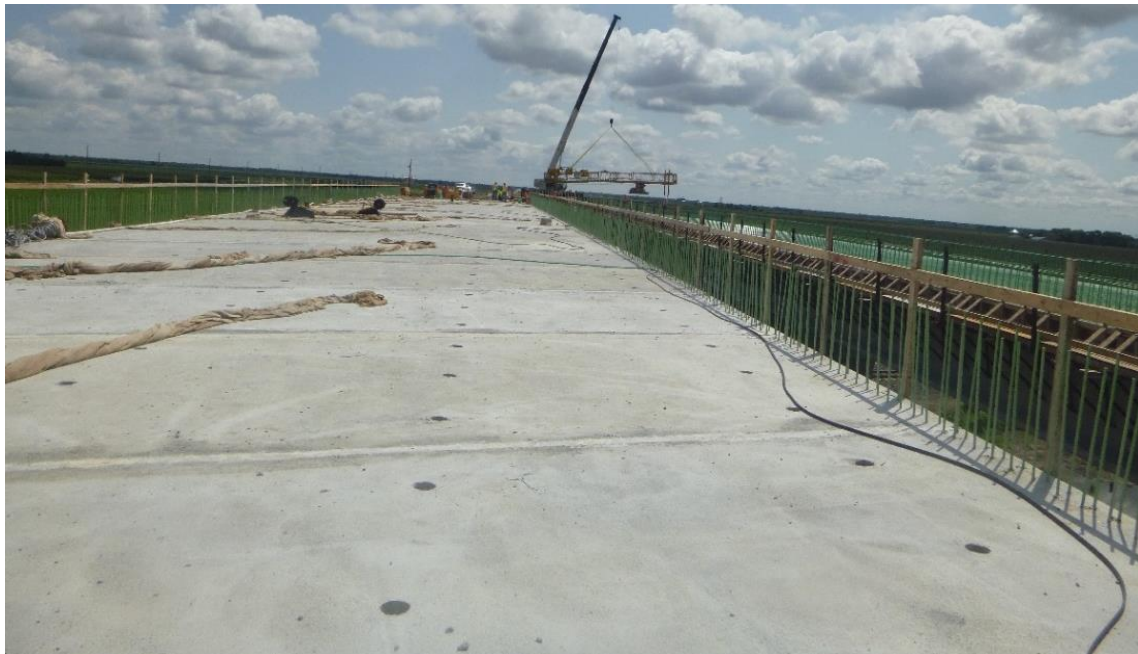
FIGURE 1.5 Precast concrete deck during and after grouting transverse joints
