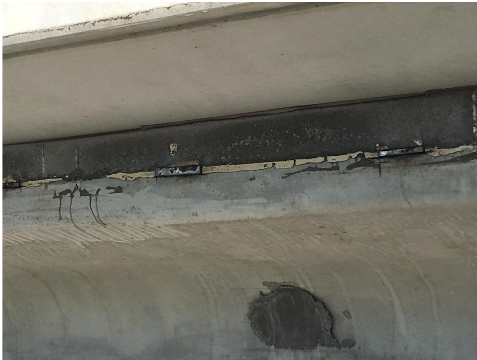
FIGURE 2.10 Exterior girder haunch cast using SCC
