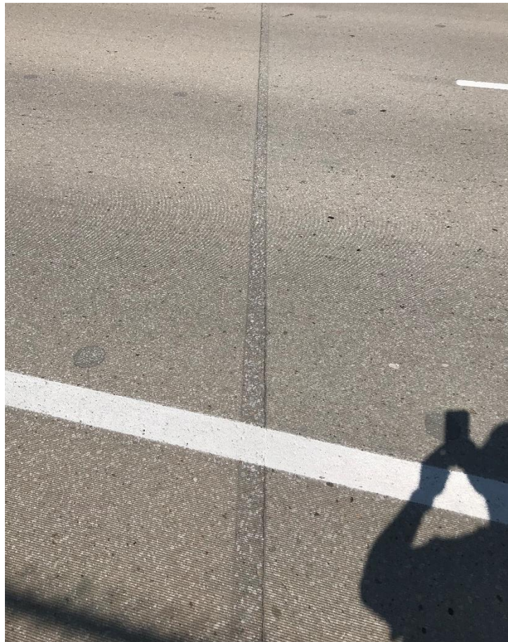
FIGURE 2.27 Pier section transverse joint in precast deck
