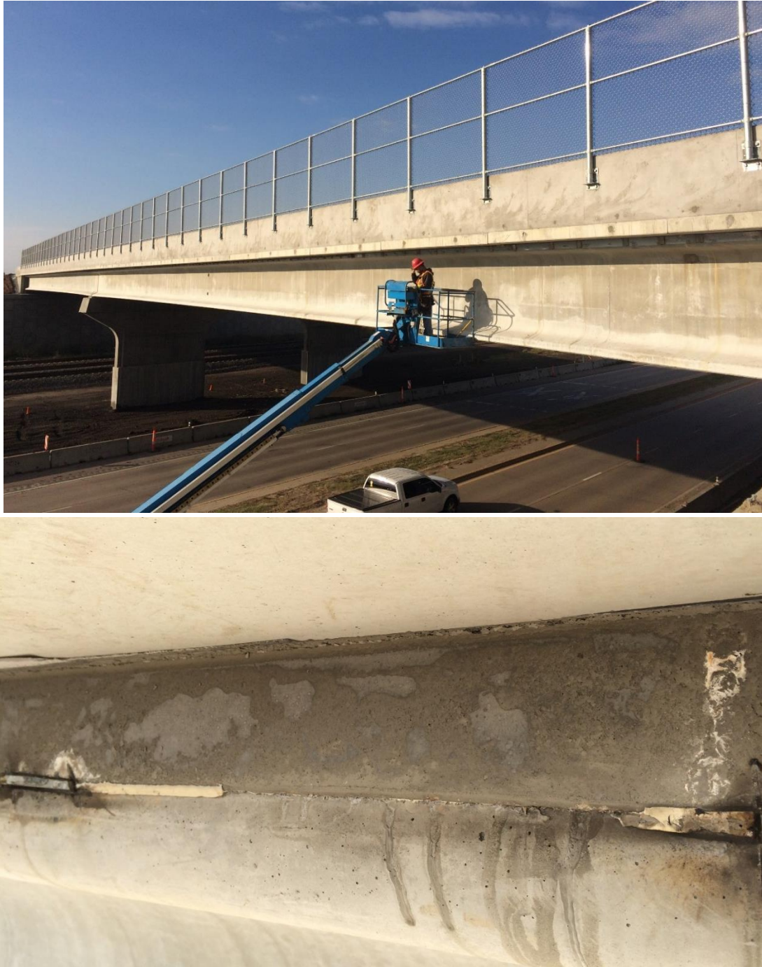
FIGURE 2.1 Removal of deck support system to inspect the SCC haunch
