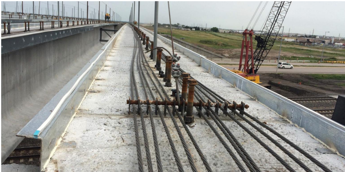
FIGURE 1.3 Deck support system, shear connectors, and PT deviators
