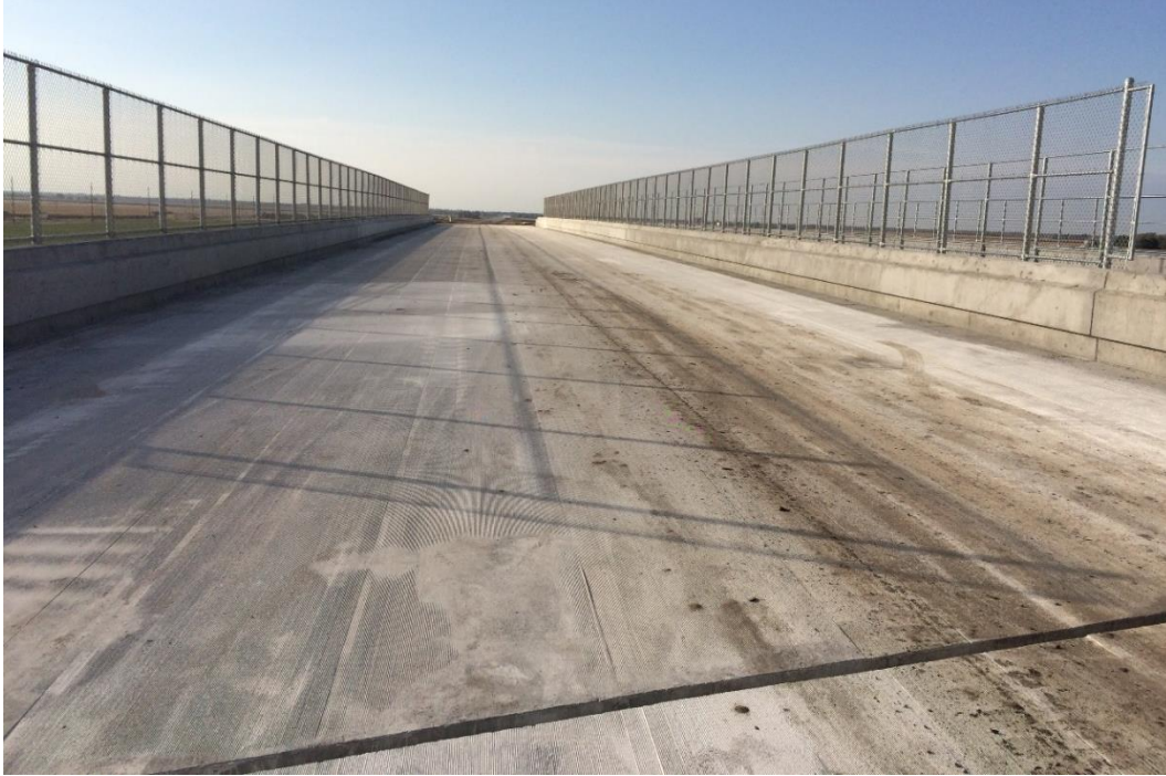
FIGURE 1.8 Precast concrete deck surface after grinding and casting the rail
