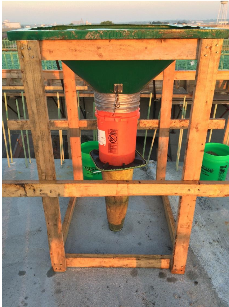
Cast-in-Place SCC for Shear Pockets and Haunches
