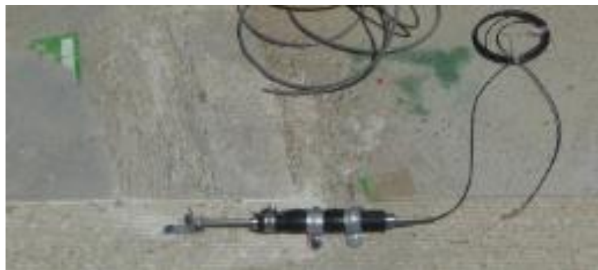
(a) LVDT installed at pier section
