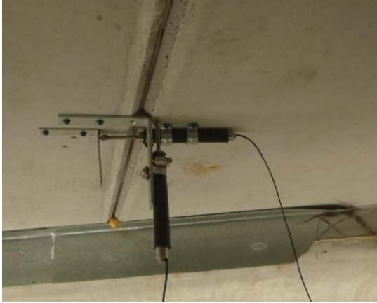
(b) LVDT installed at pier section
