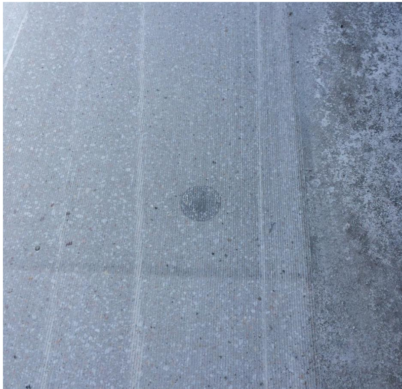
FIGURE 2.3 Grouting hole in precast concrete deck panels
