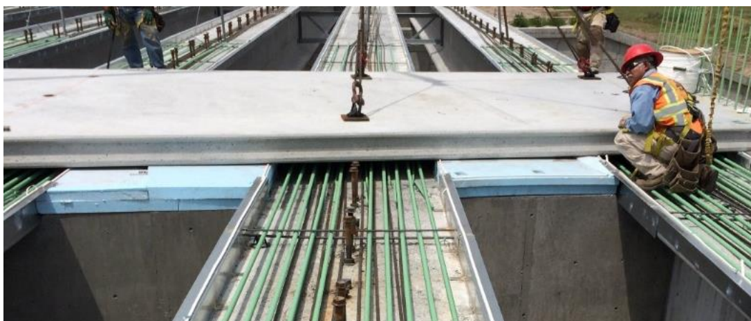
FIGURE 1.4 Deck panel erection
