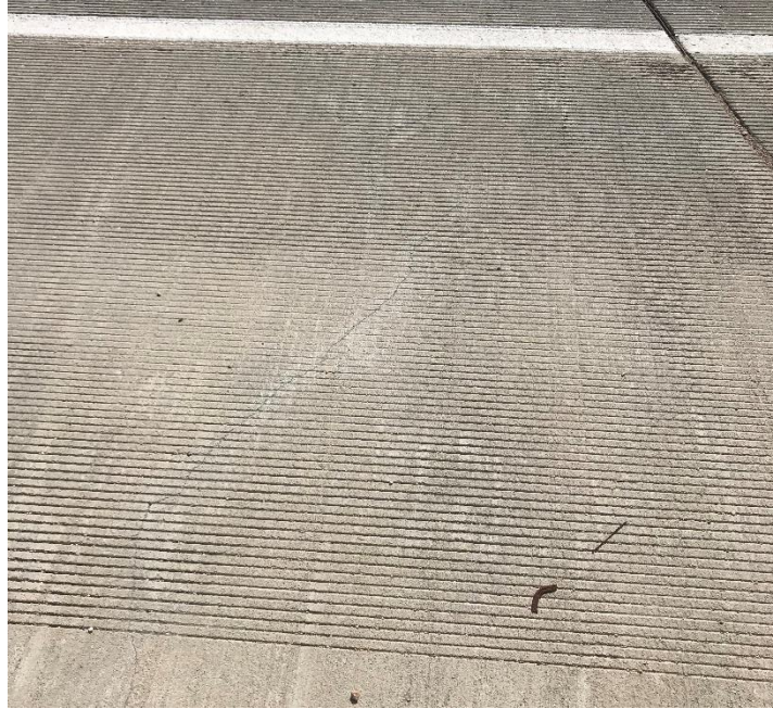
FIGURE 2.26 One of the transverse cracks extending the full width of CIP deck
