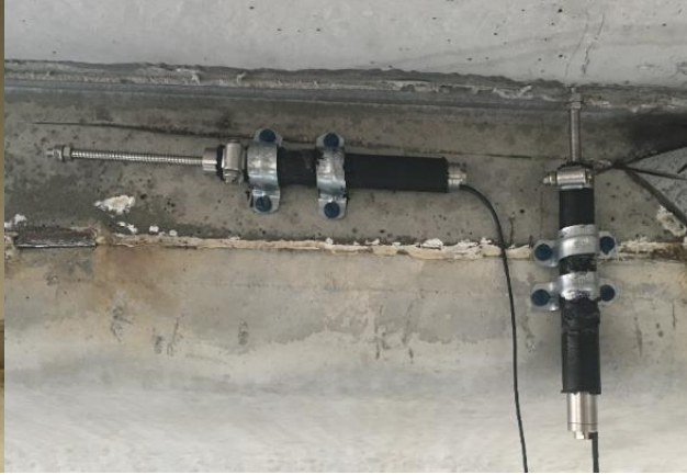
(c) LVDT installed at pier section
