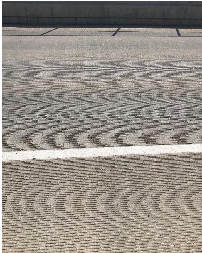
FIGURE 2.25 Multiple transverse cracks at the negative moment region of CIP deck
