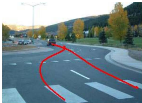
Figure 1.4 Insufficient entry path (Source: Safety Auditing Roundabouts 2004)
