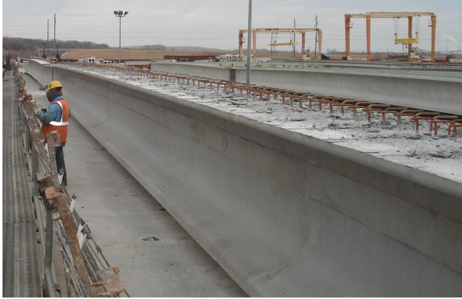
Figure 8: Camber of the 140 ft long girders at release
