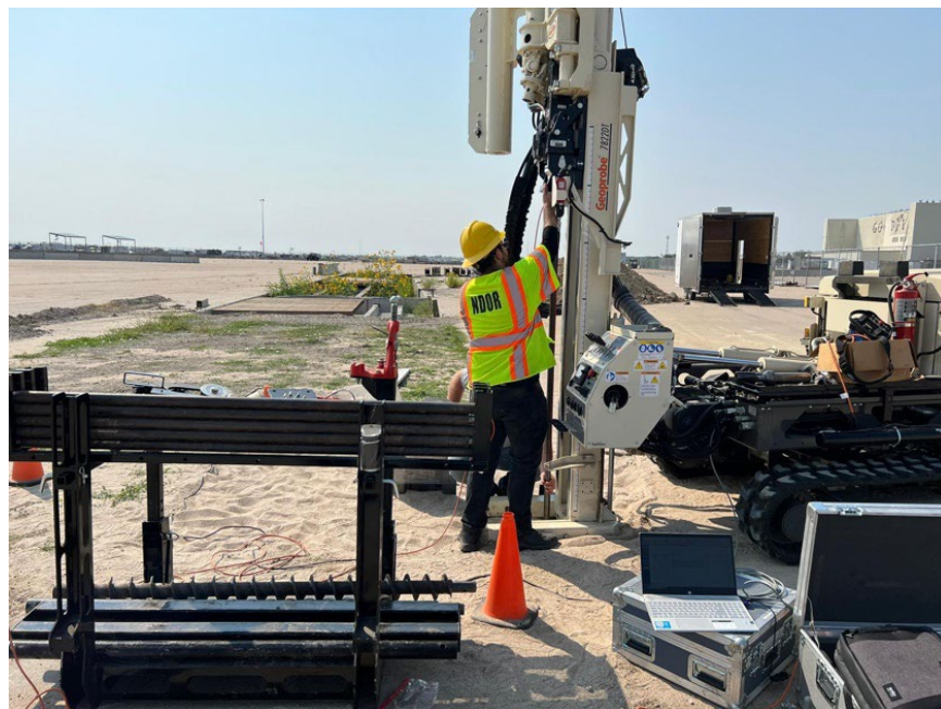
Figure 4.13 CPT test conducted by the research team.
