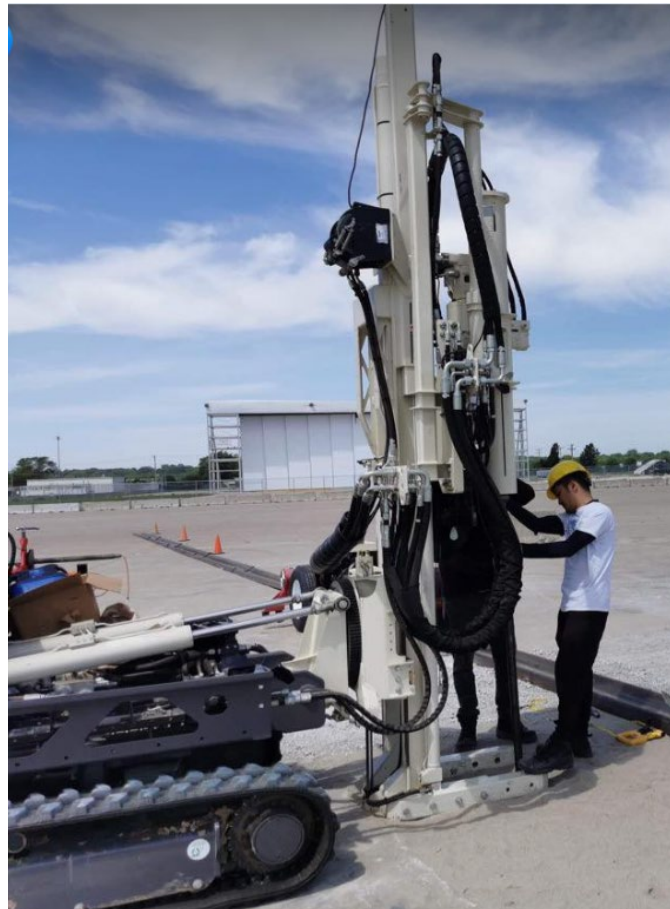
Figure 4.9 Geoprobe 7822 DT used for the subsurface investigation of the test site.
