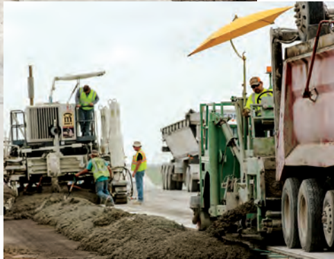
Paving work on Hwy. 385 south of Alliance
