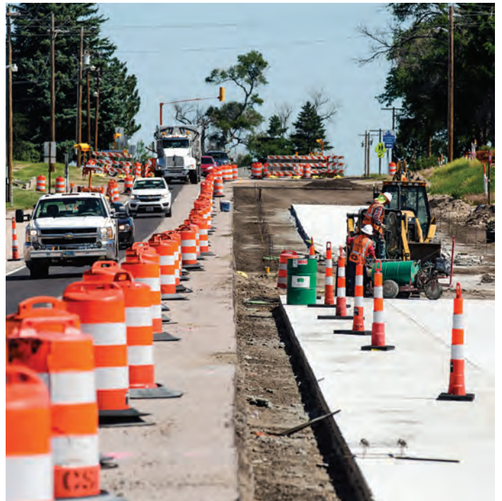
Construction on Hwy. 385 near Dalton
