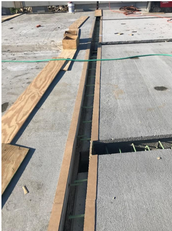
End of Floor Connection
