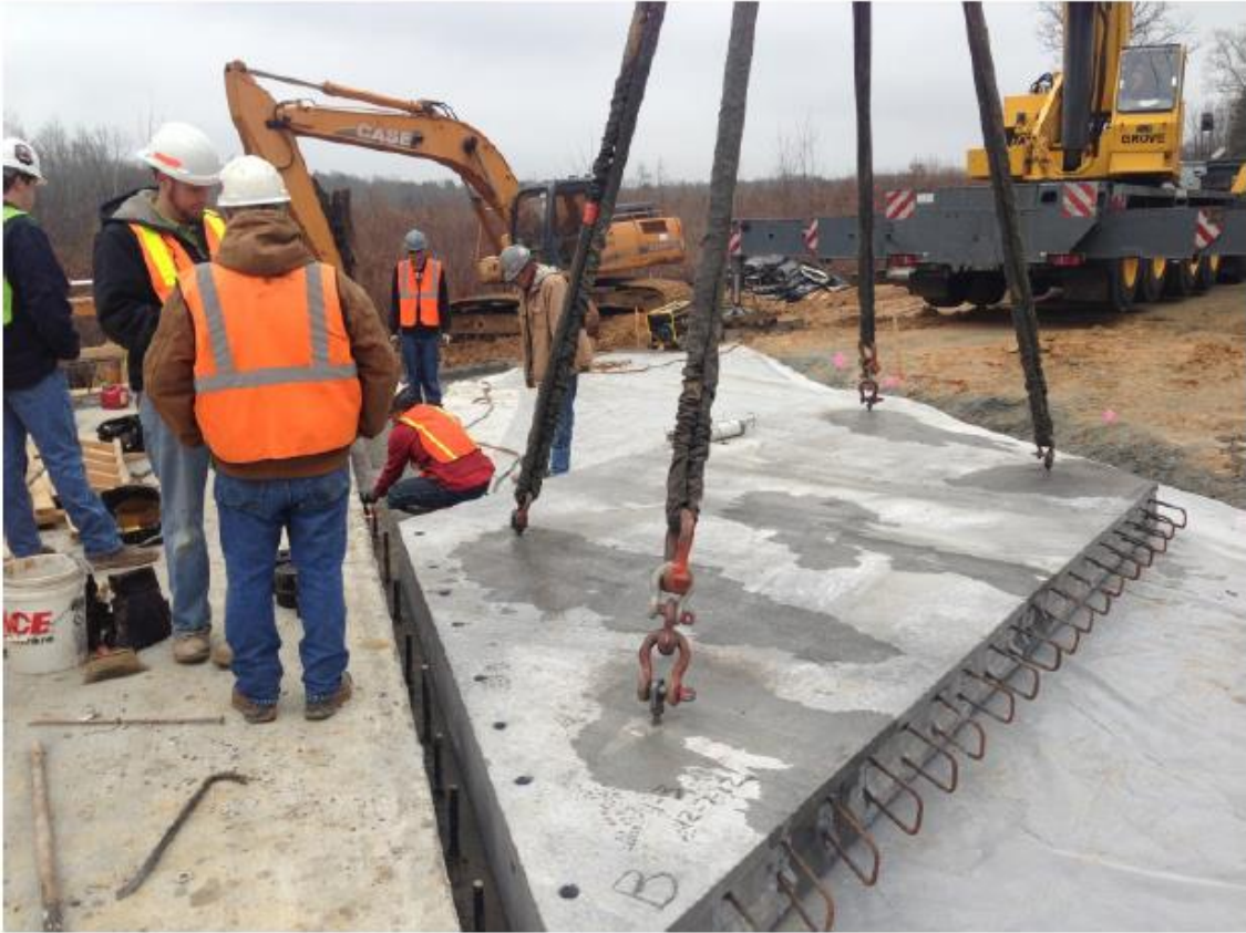
Panel installation over polyethylene sheeting
