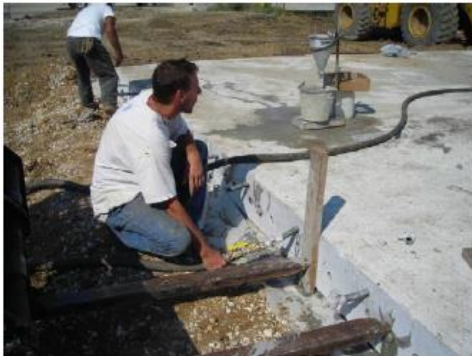
Grouting underneath the precast panels
