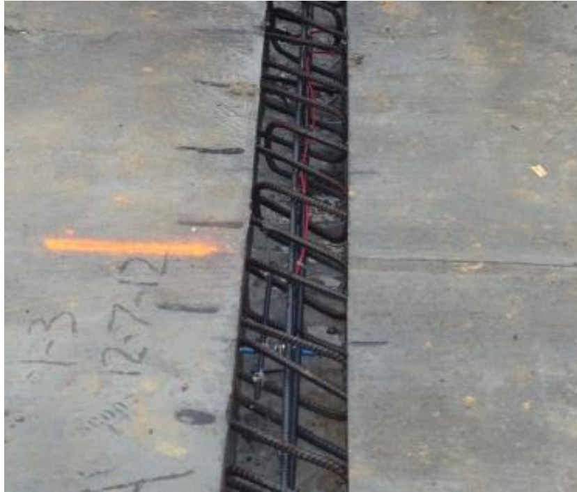
Reinforcement of longitudinal joints
