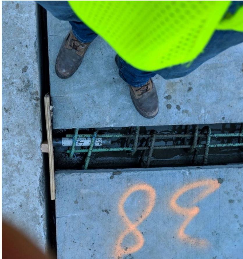
Precast panel joints and connections
