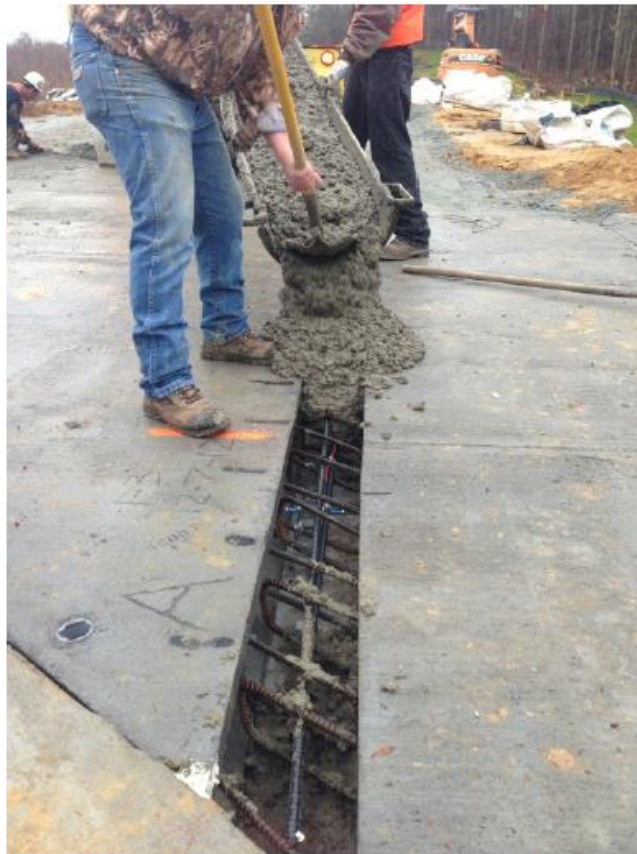
Casting longitudinal joints
