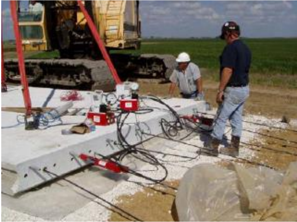
Stressing longitudinal post-tensioning strands
