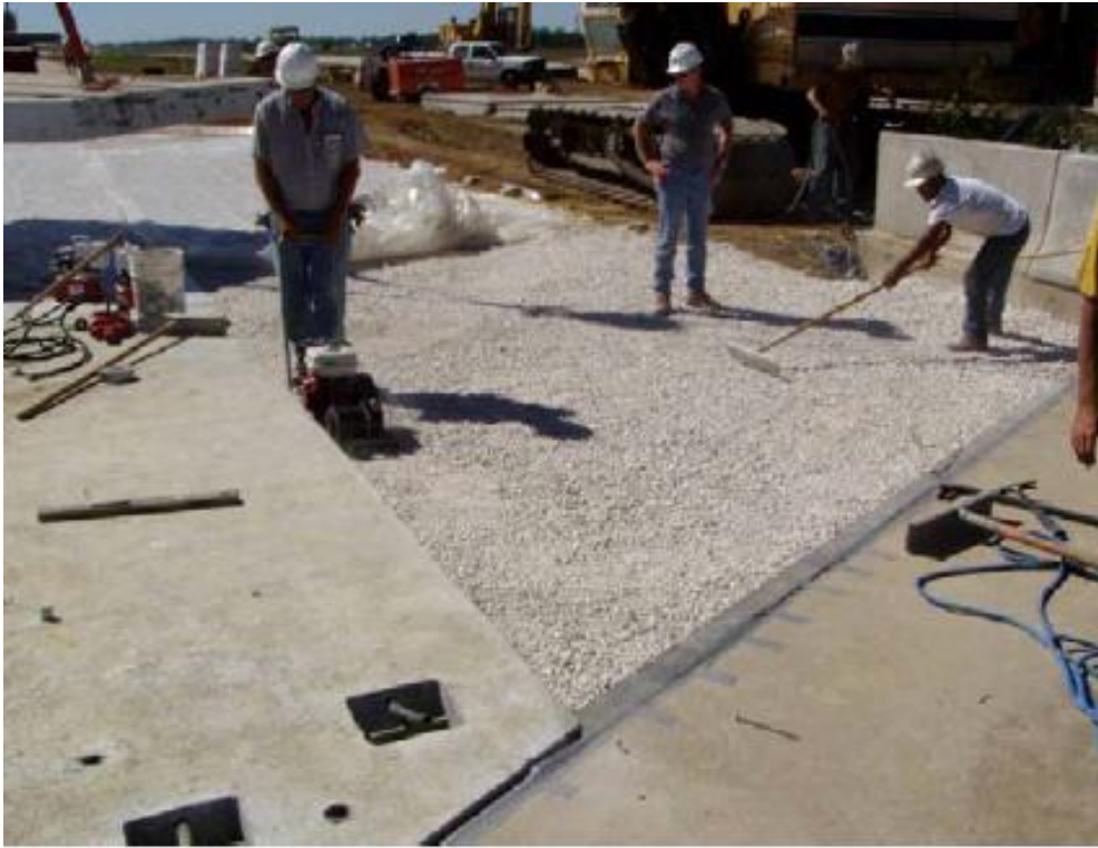
Panel base preparation
