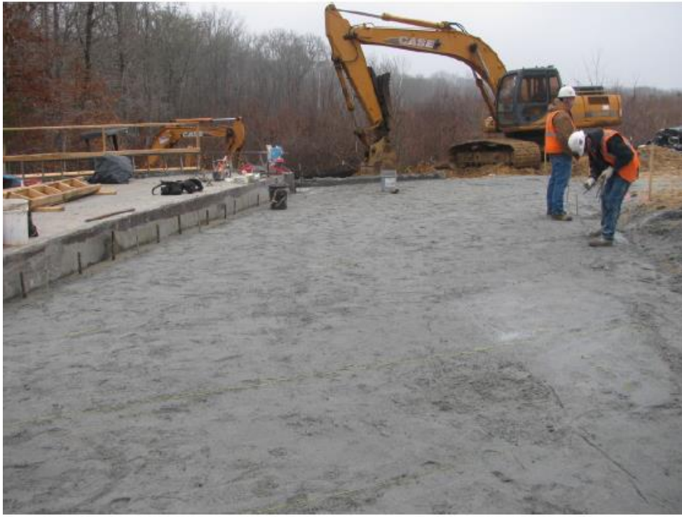
Panel base preparation
