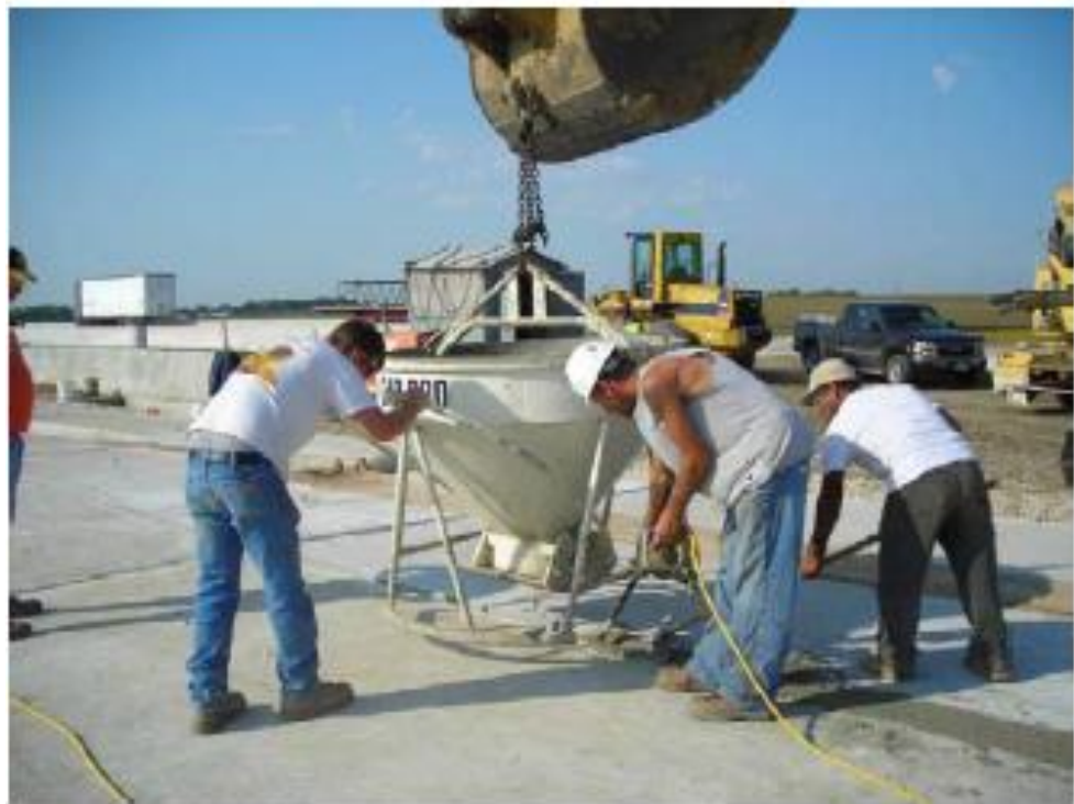
Casting longitudinal joint
