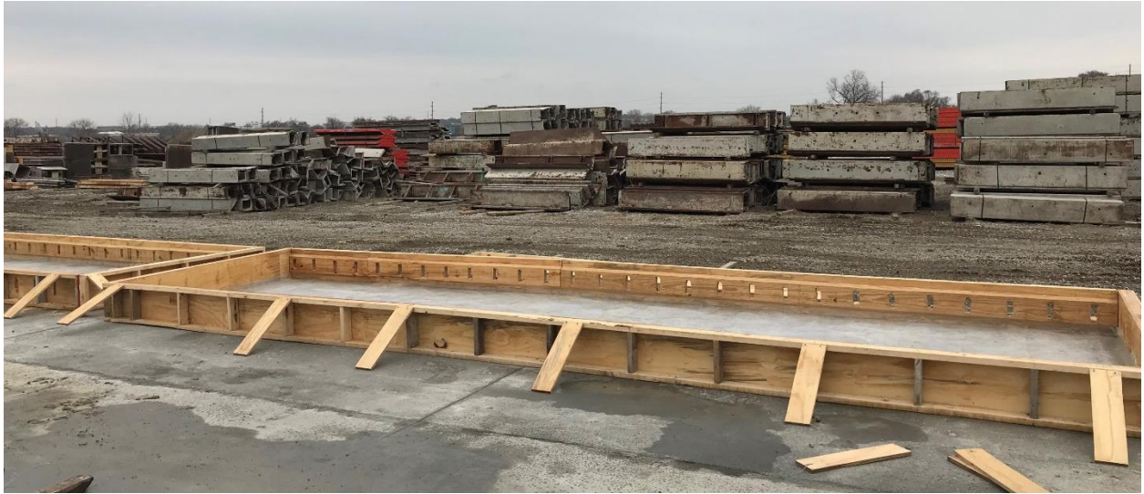
Forming paving section panels
