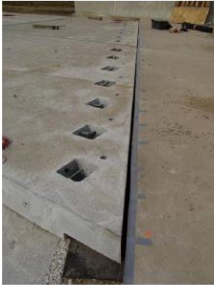
Matching panels at the end of floor
