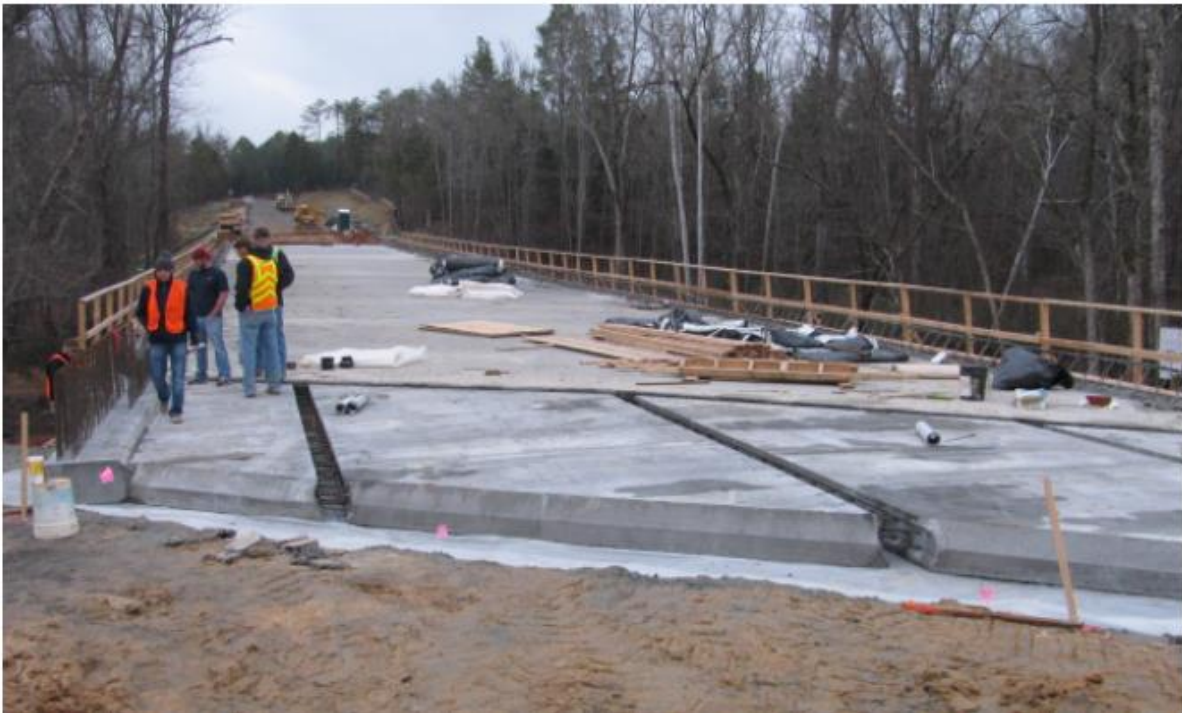
Complete installation of skewed panels
