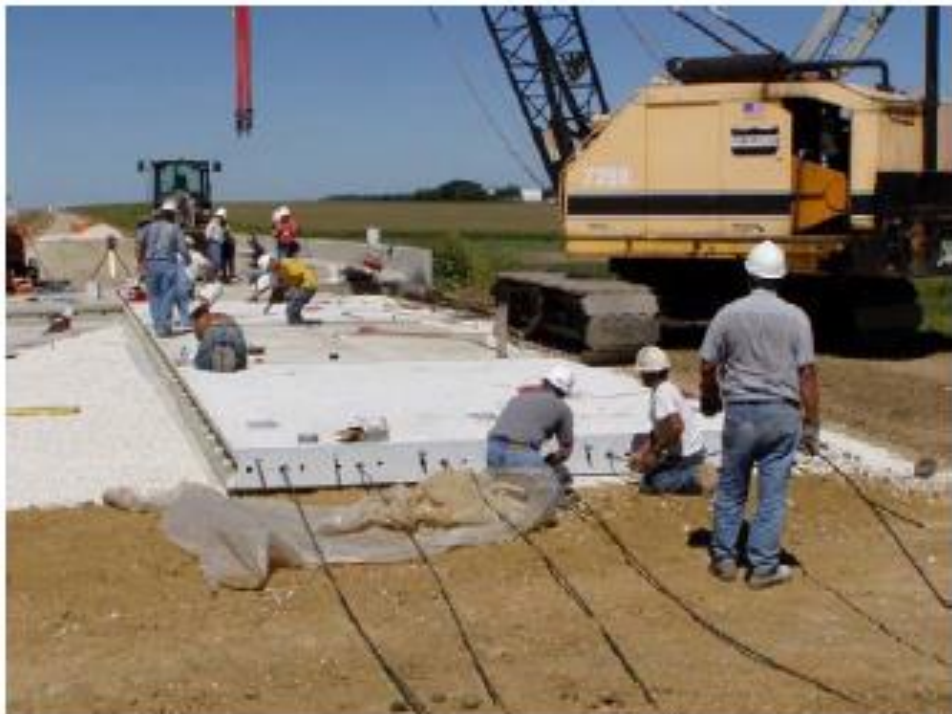
Threading longitudinal post-tensioning strands
