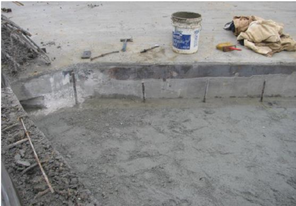
Vertical dowels for the end of floor connection
