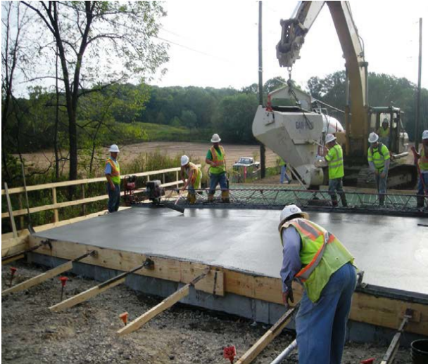
Figure 14. Internally cured bridge deck placed by means of a bucket
