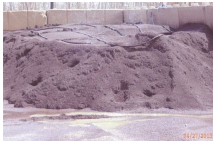
Figure 18. LWA piles being soaked prior to batching of internally cured concrete
