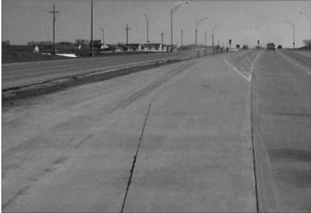
Figure 11.4 Gravel-Cleared Paths on Offset Left-Turn Lanes
