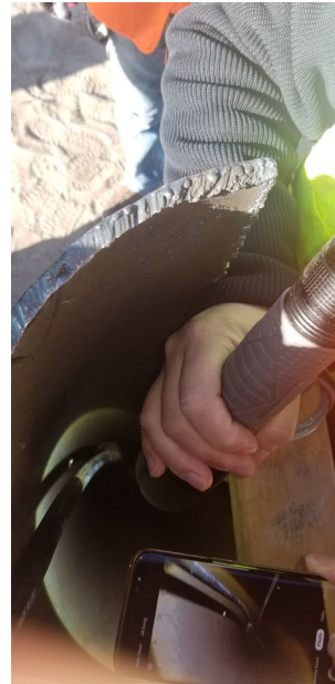
Figure 3.35 Lowering the composite beams into the pile
