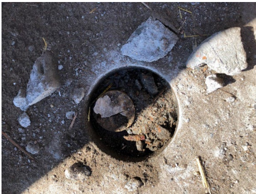
Figure 3.28 Inclinator Casings after Cutting Open the Approach Slab
