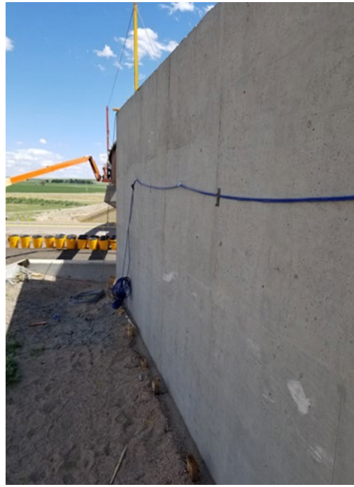
(a) channeling out the pressure cell cables (b) securing them behind the wingwalls
