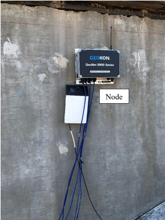
Figure 3.45: Photo of Solar Panel, the Node and the Supervisor on both Abutments
