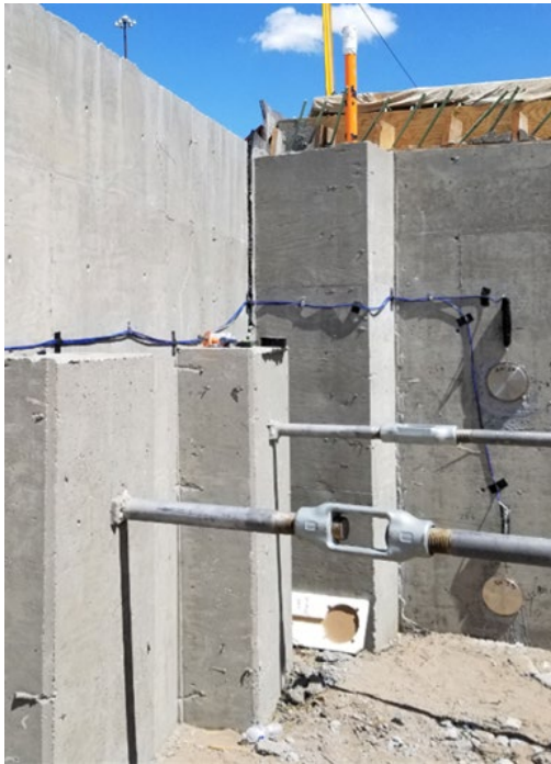
(a) channeling out the pressure cell cables (b) securing them behind the wingwalls
