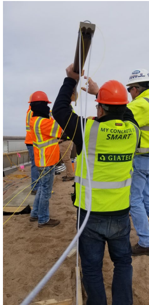
Figure 3.35 Lowering the composite beams into the pile
