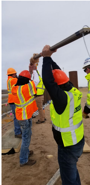
Figure 3.35 Lowering the composite beams into the pile
