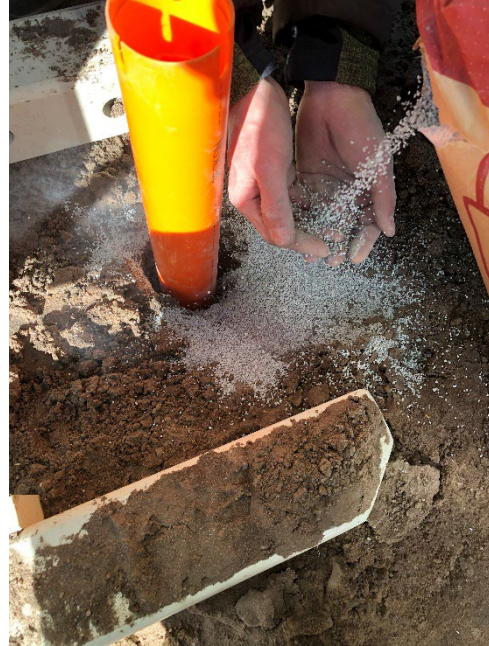
(b) filling the gap with bentonite
