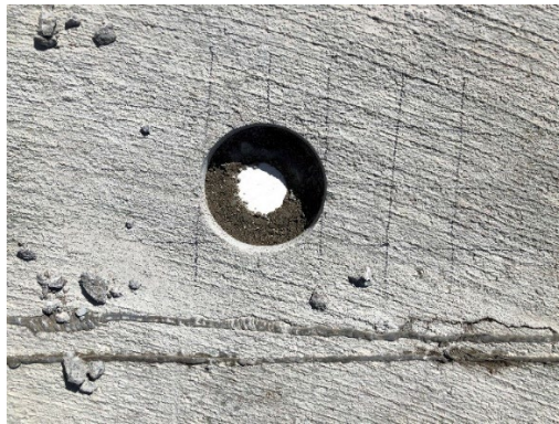
Figure 3.28 Inclinator Casings after Cutting Open the Approach Slab
