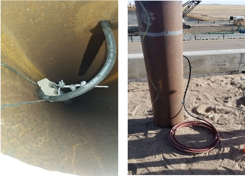
Figure 3.36: Rubber Tube Installation for Cable Protection
