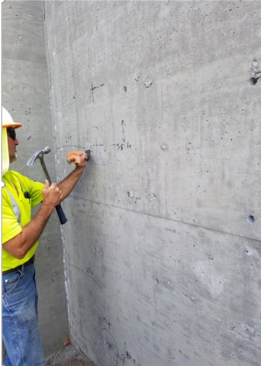
(a) cleaning and leveling the installation location
