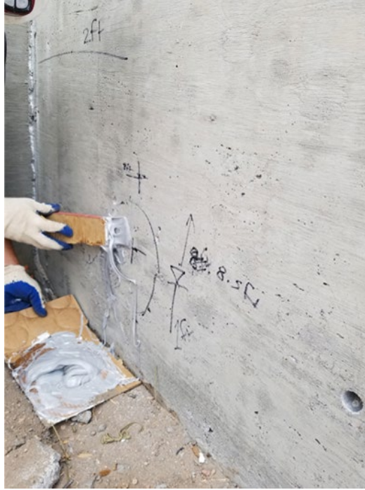
Figure 3.9: Adding Epoxy to the Contact Area to Secure the Installation
