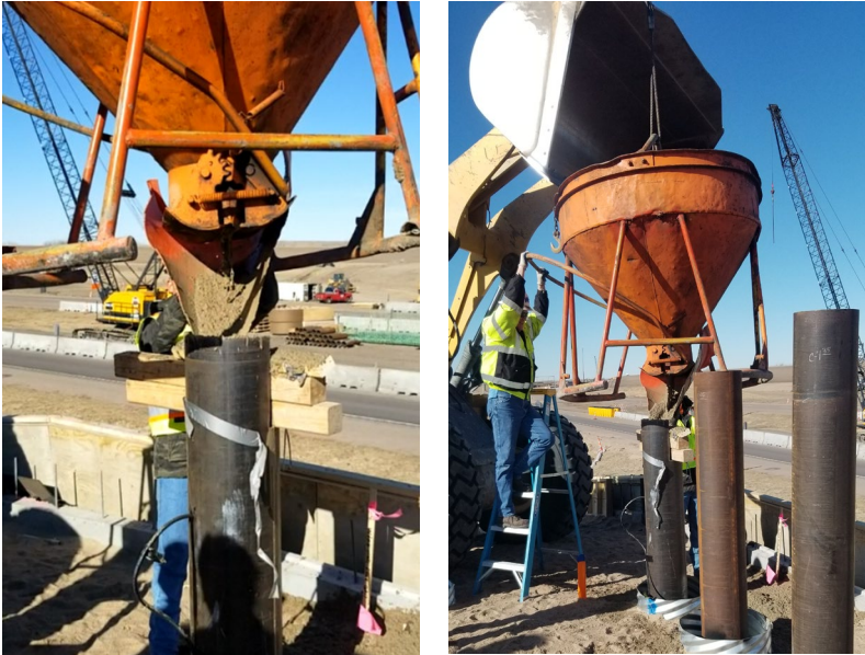
Figure 3.37: Casting Mortar inside Piles with Fiber Optic Cables
