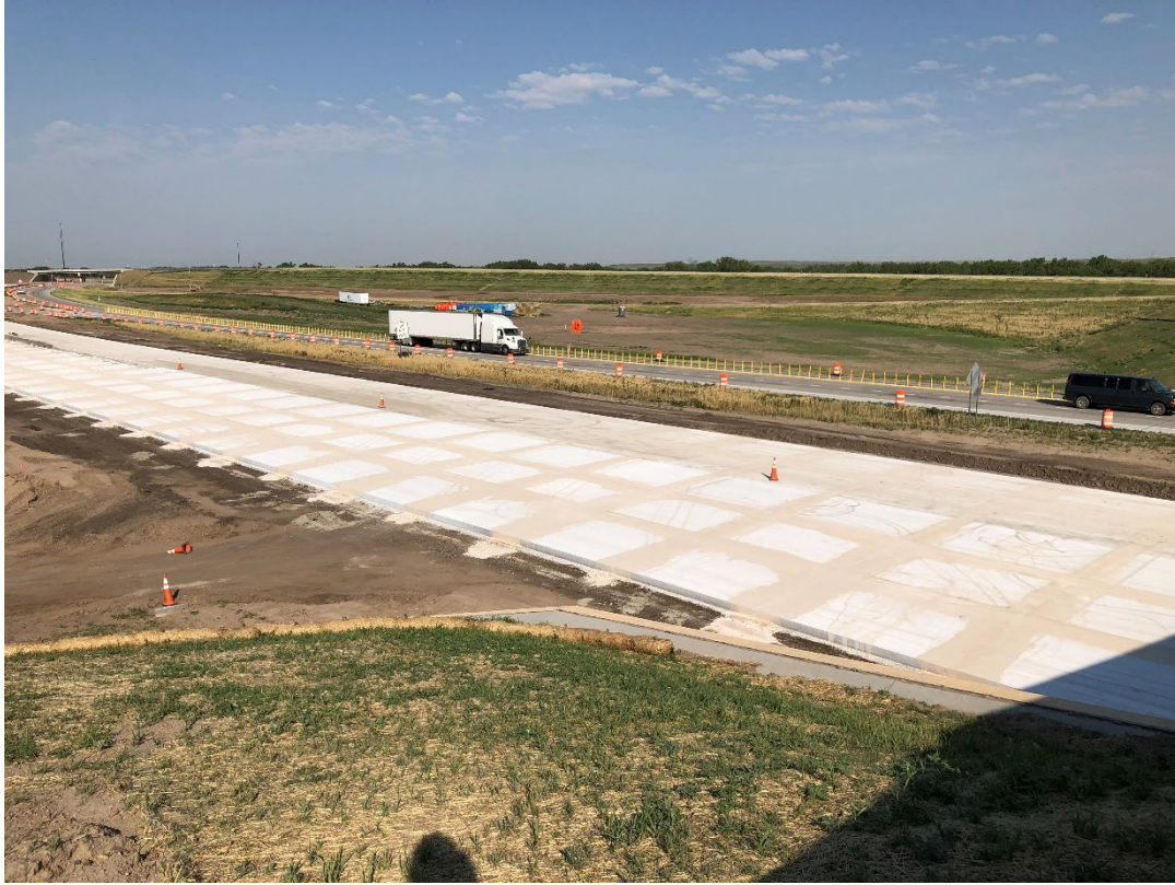
Figure 3.2: Pavement Replacement as Part of the Big Springs West Project
