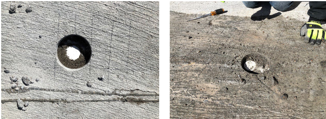
Figure 3.26: Cut Open Section near Approximate Location of the Inclinometer Casing
