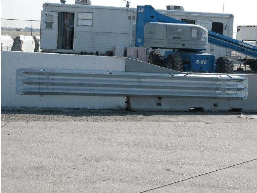
Figure 11. Transition from PCB to Permanent Concrete Barrier [2]
