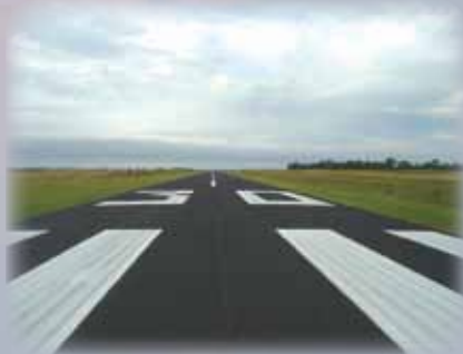
Runway Seal Coat and Marking
