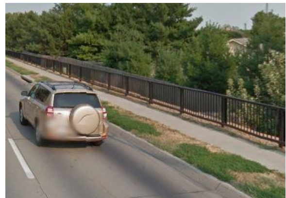
Figure 2.6 Examples of Safety Railings between Trails/Sidewalks and Watercourses/Retaining Walls
