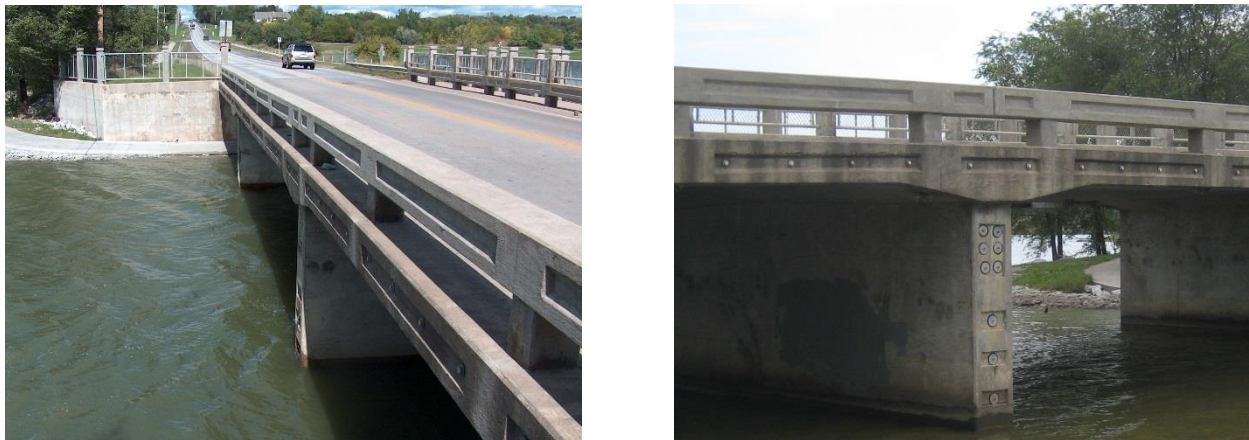
Figure 1.6 Existing Zorinsky Lake Bridge Conditions
