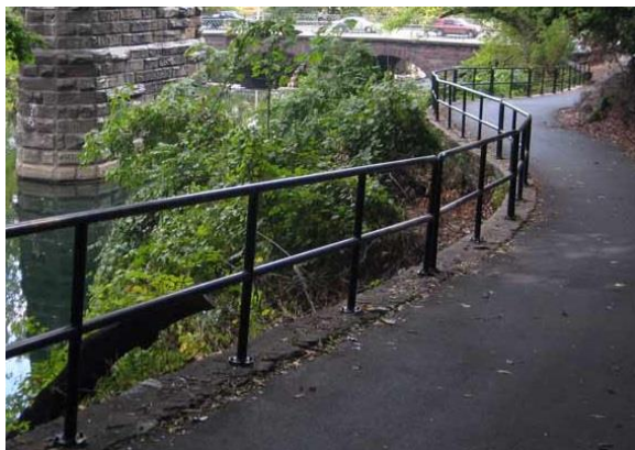
Figure 2.6 Examples of Safety Railings between Trails/Sidewalks and Watercourses/Retaining Walls
