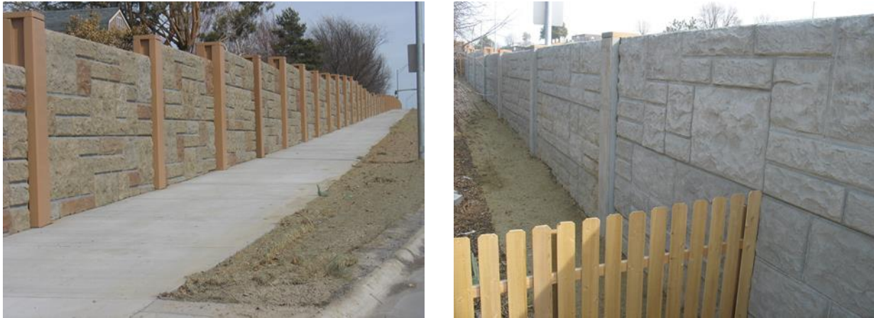
Figure 3.20 Typical Noise Walls
