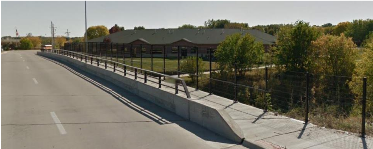
Figure 2.5 Example of Proposed Bridge Railing System
