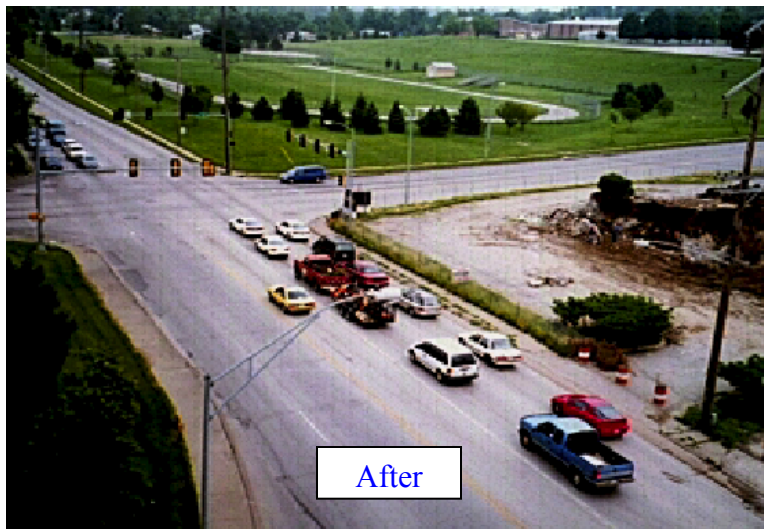
Figure 3.6. Before and After Left-Turn Lane Lines at 72 nd and Cass St.
