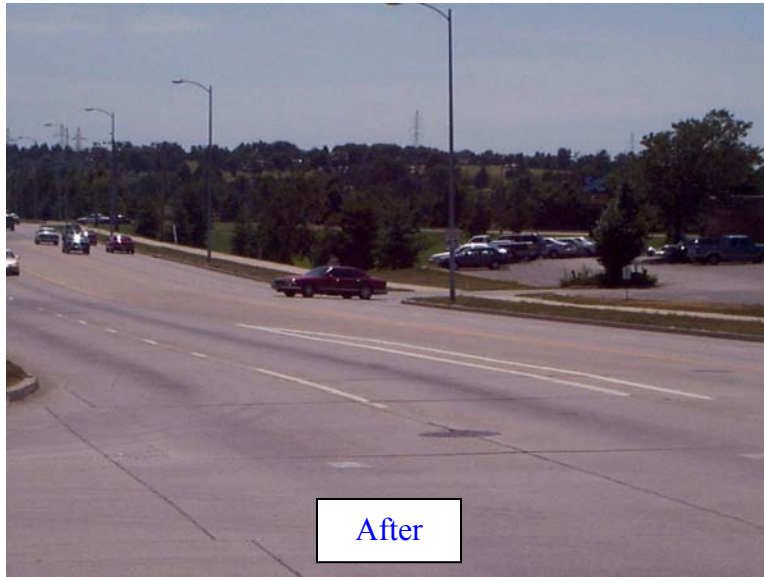
Figure 3.2. Before and After Left-Turn Lane Lines at 70 th and Van Dorn St.
