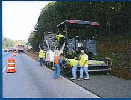
New Concrete Placed
