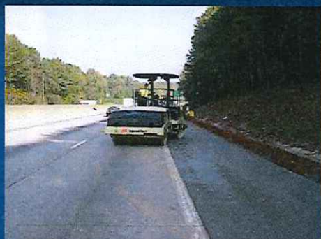
Initial Roller Compaction
