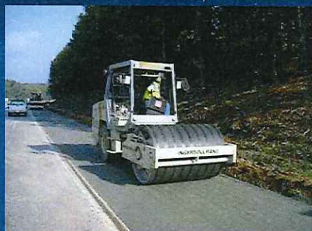
Roller Compaction (rubber-coated drum)
