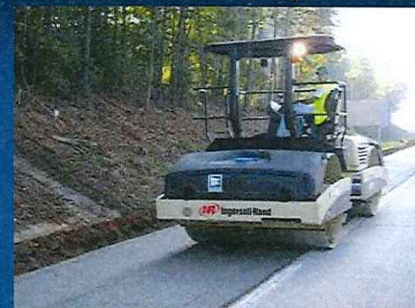
Initial Roller Compaction
