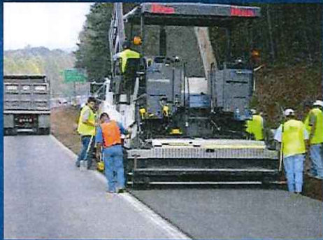
New Concrete Placed
