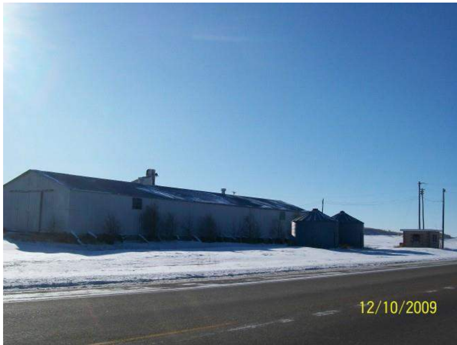
Figure 4. View of FN2015-02, steel storage bridge, steel grain bins and concrete block scale house. Morrill County Assessor photo.
