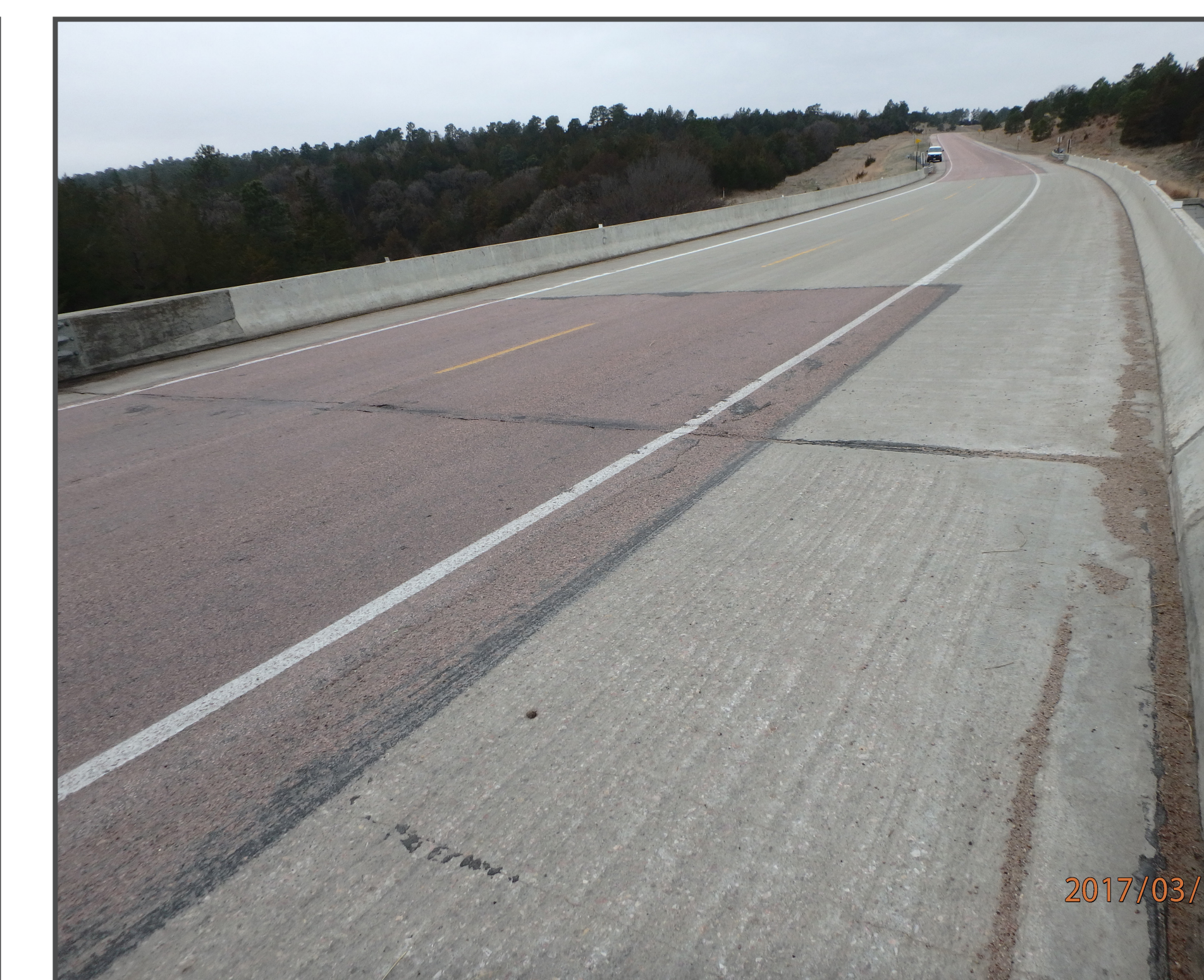
Approach slab and bridge surface looking west
