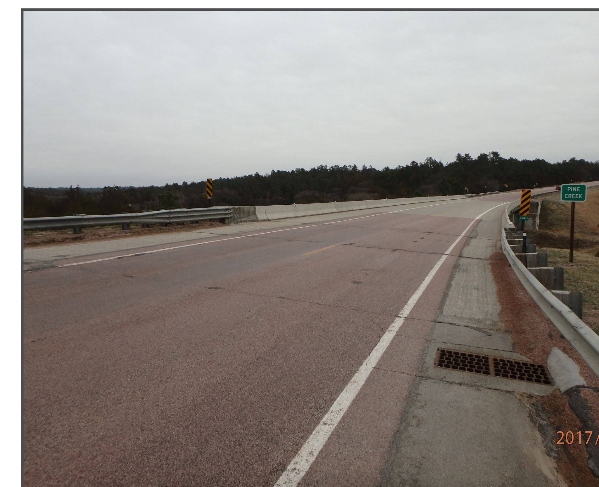
Approach slab and bridge surface looking east
