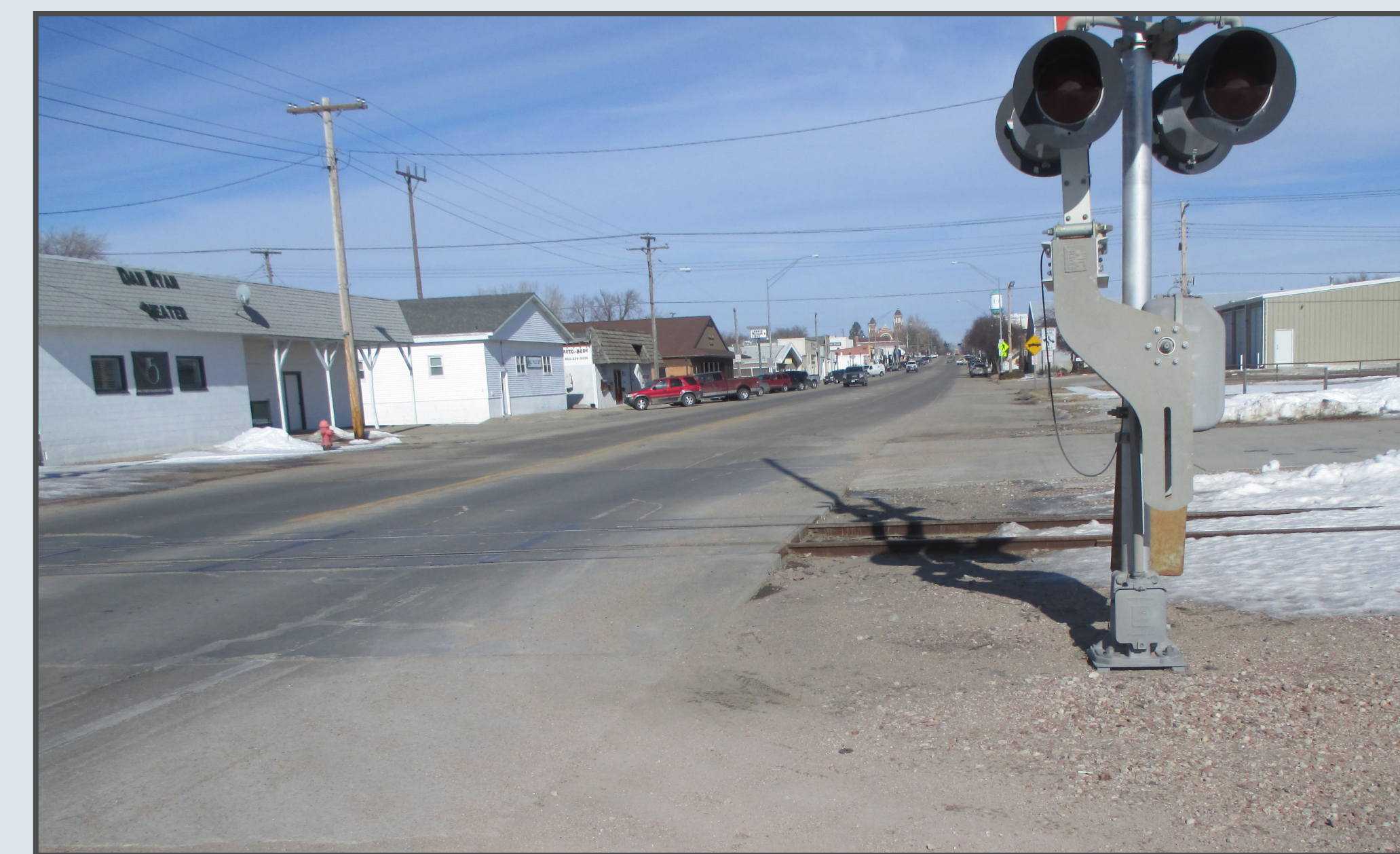
The railroad crossing signals would be removed and replaced.
