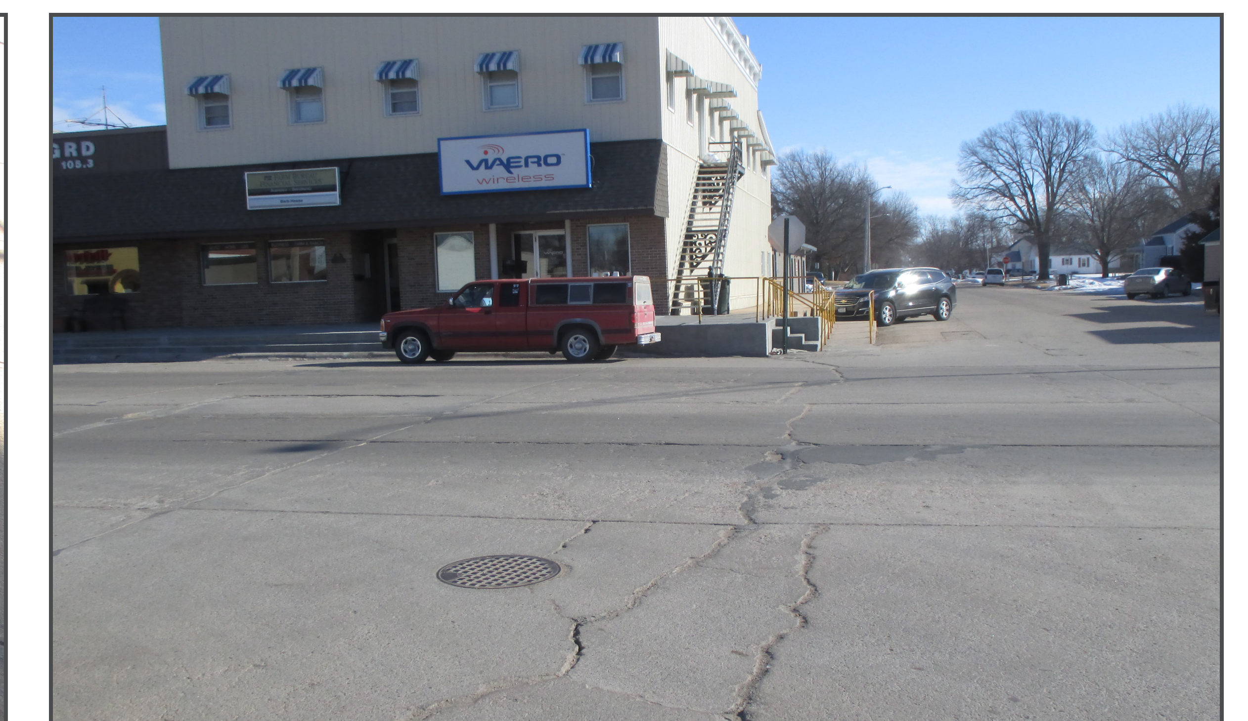
Deteriorating sidewalk (left) and roadway pavement (right) can be seen throughout the project area.
