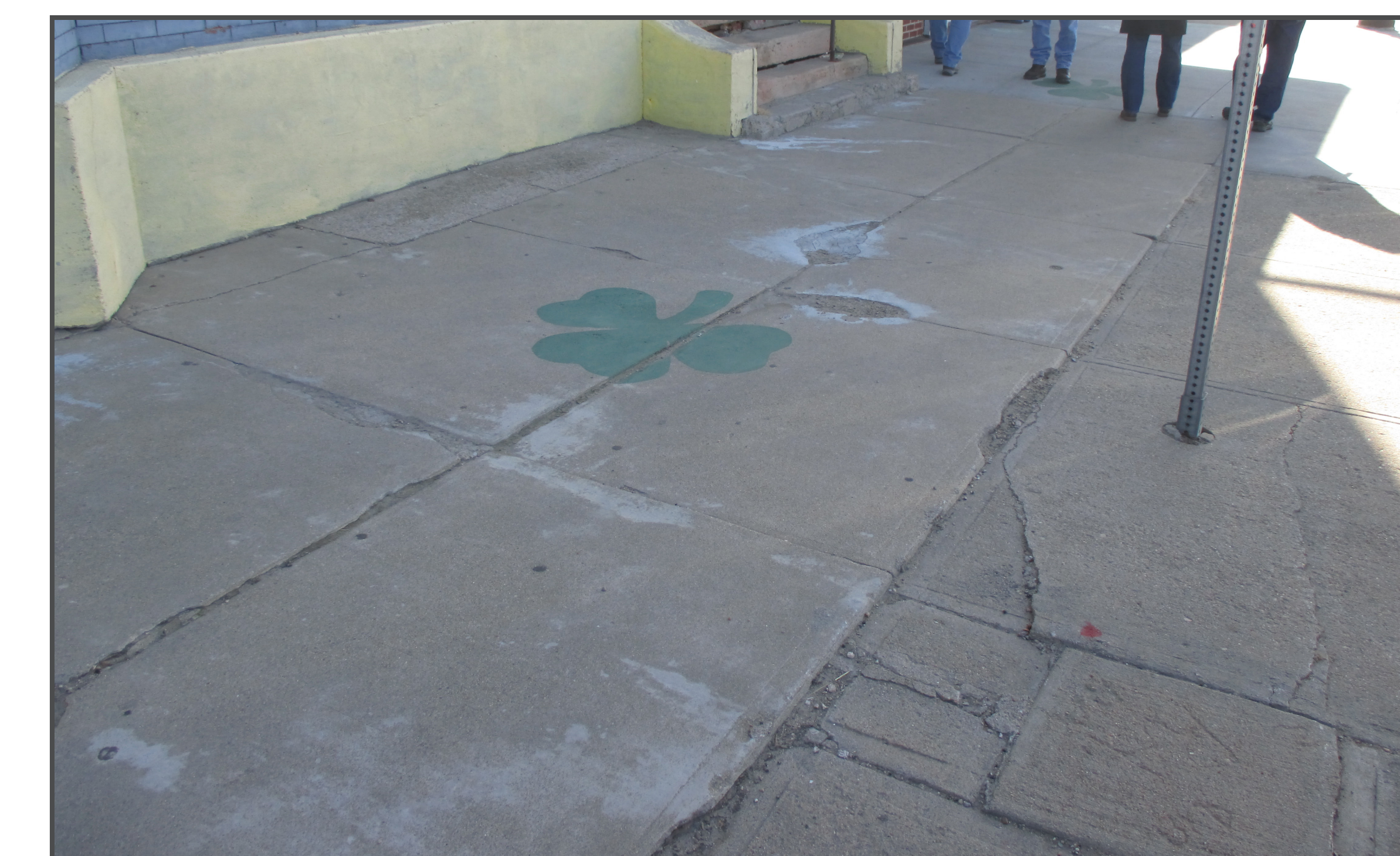
Deteriorating sidewalk (left) and roadway pavement (right) can be seen throughout the project area.
